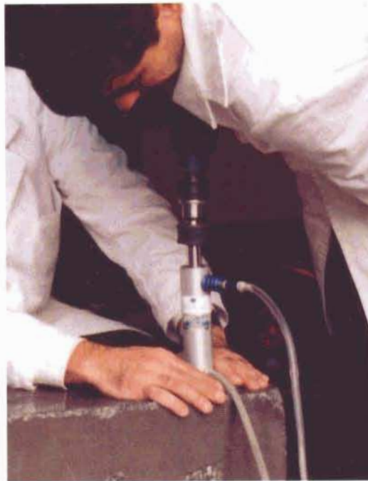
Figure 5 - Drilling a 18 mm centre hole with a drill unit.
