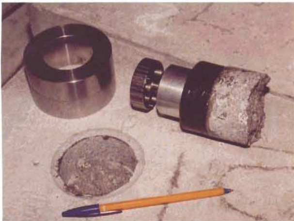
Figure 13 - Failure type is observed for validation of result.
