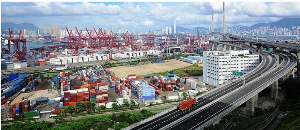
Fig. 2 - Hong Kong, Porto de Kwai Chung.
