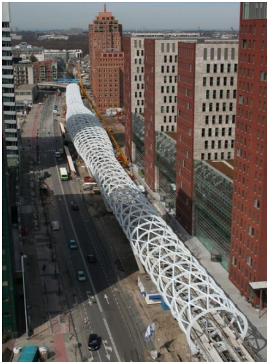
Fig. 31- Light-rail station, vista aérea
