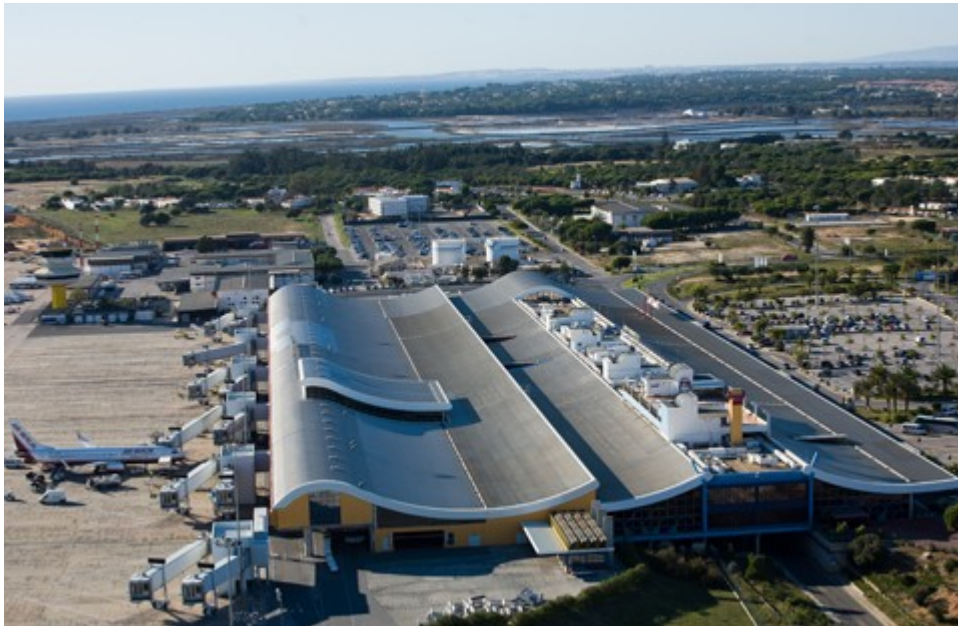
4.70: Faro Airport (Zagope, 2012)
