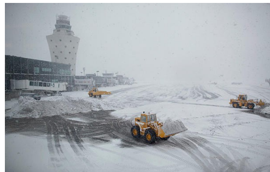
Figure 2.13: Works on Snow Removal at La Guardia airport, New York City, during December 2010 Snowstorms (CSmonitor.com, 2012)
