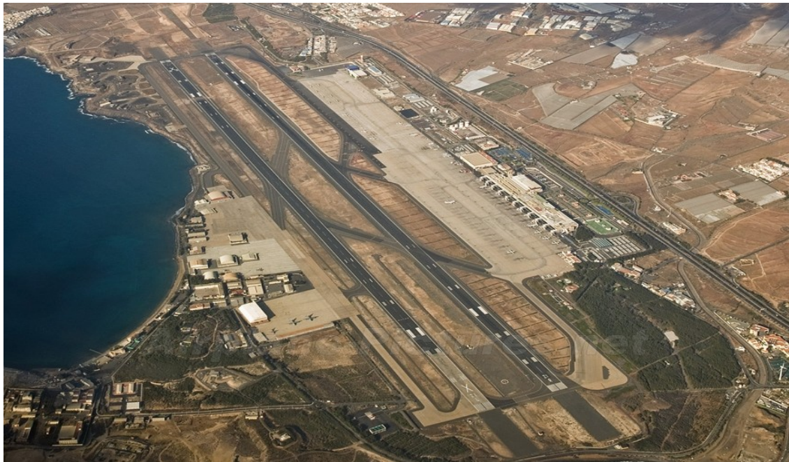
Figure 4.136: Gran Canaria Airport (Heijst, 2012)
