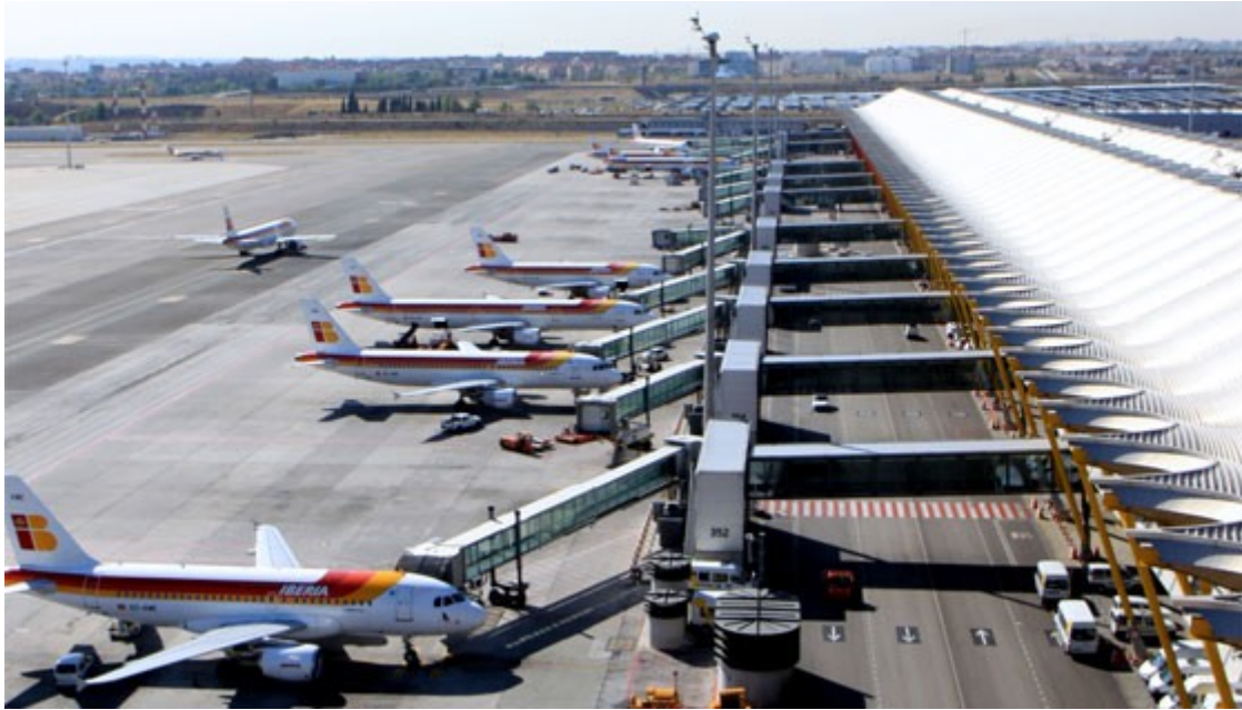
Figure 4.103: Madrid Barajas Airport Terminal 4 (AENA, 2012a)
