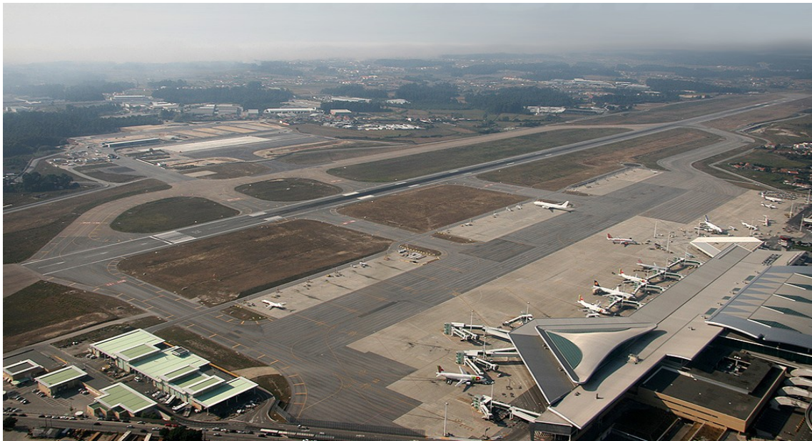
Figure 4.59: Porto Airport (Resendes, 2012)
