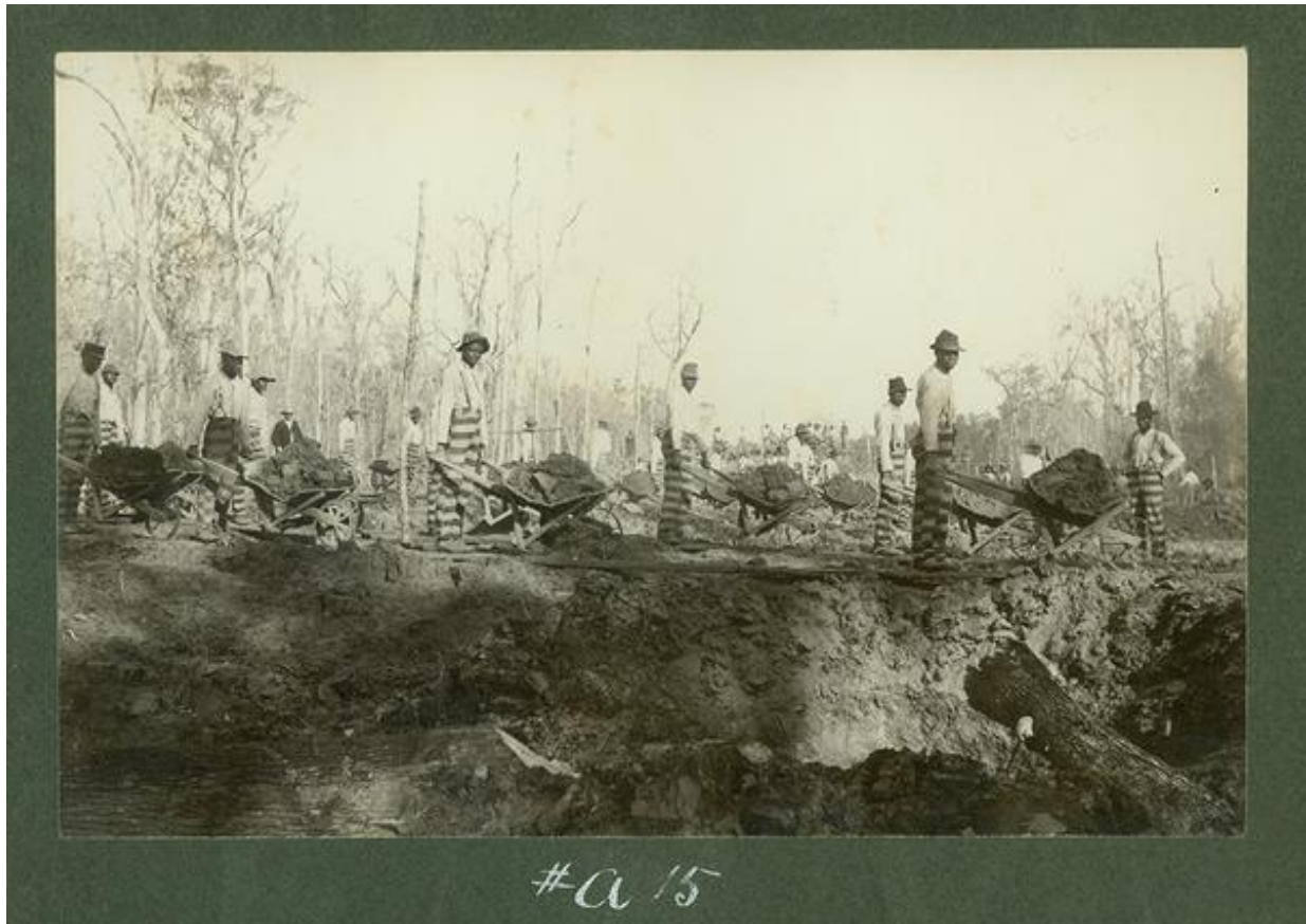
Figure 3. Convict labor at work on a levee along the Atchafalaya River, circa 1899. 112
