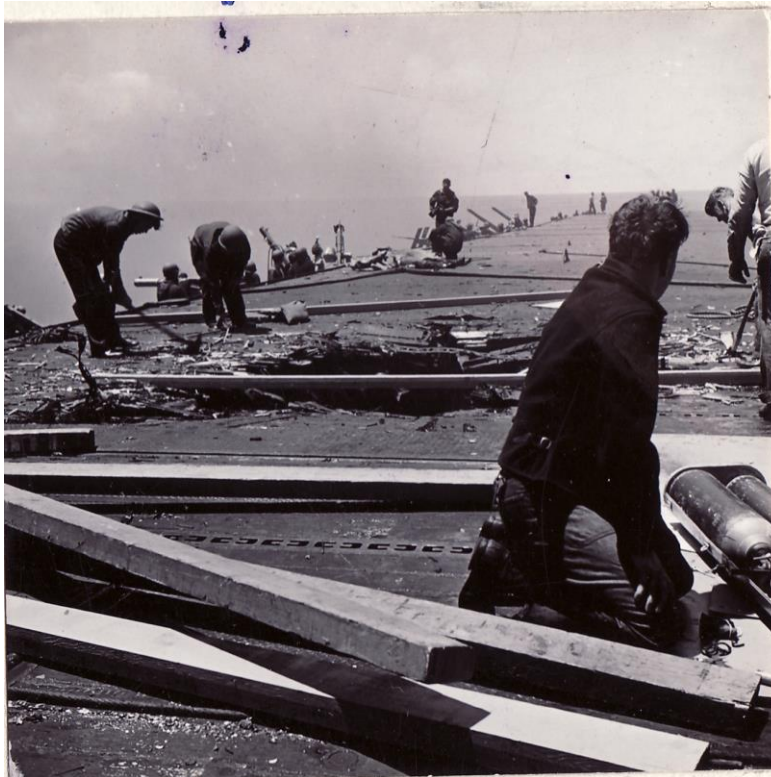
Figure 1- Damage Control repairs CV 5 flight deck at Midway (from The National World War II Museum)
