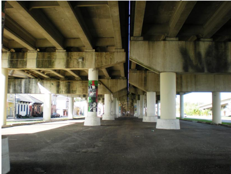
Figure 5.15 – North Claiborne Avenue at Dumaine Street (looking east), 2012. 98
