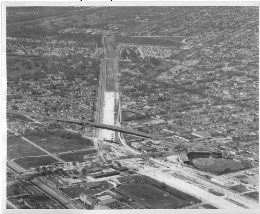
Figure 5.1 – Photograph of the Filled New Basin Canal Illustrating the Available Right-of-Way to be used for the Pontchartrain Expressway. 30
