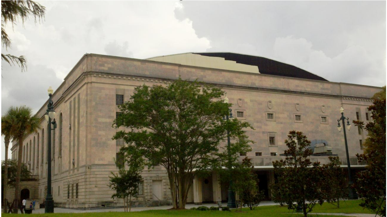
Figure 2.6 – Current Condition of the Municipal Auditorium 83
