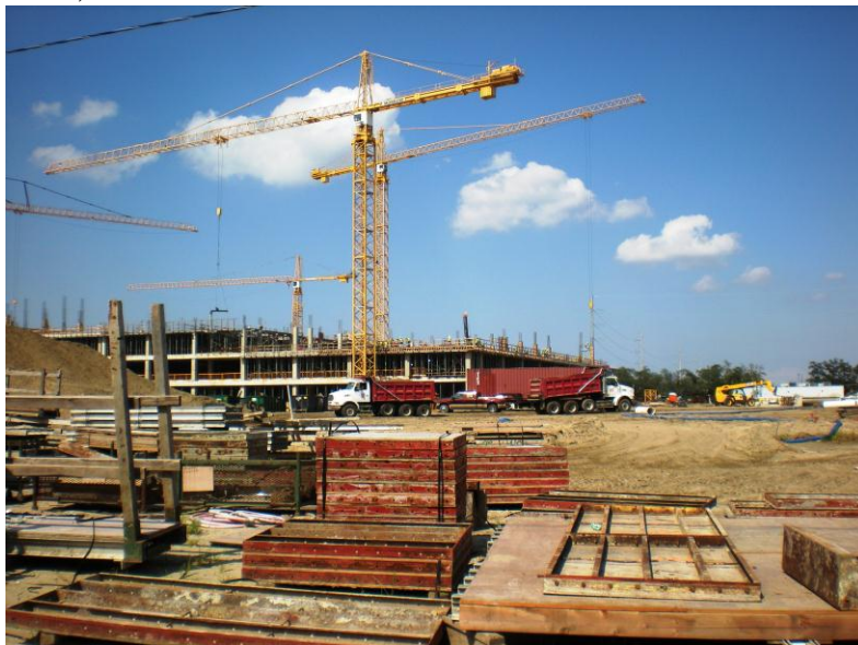
Figure 7.13 – MCLNO, under construction. 95
