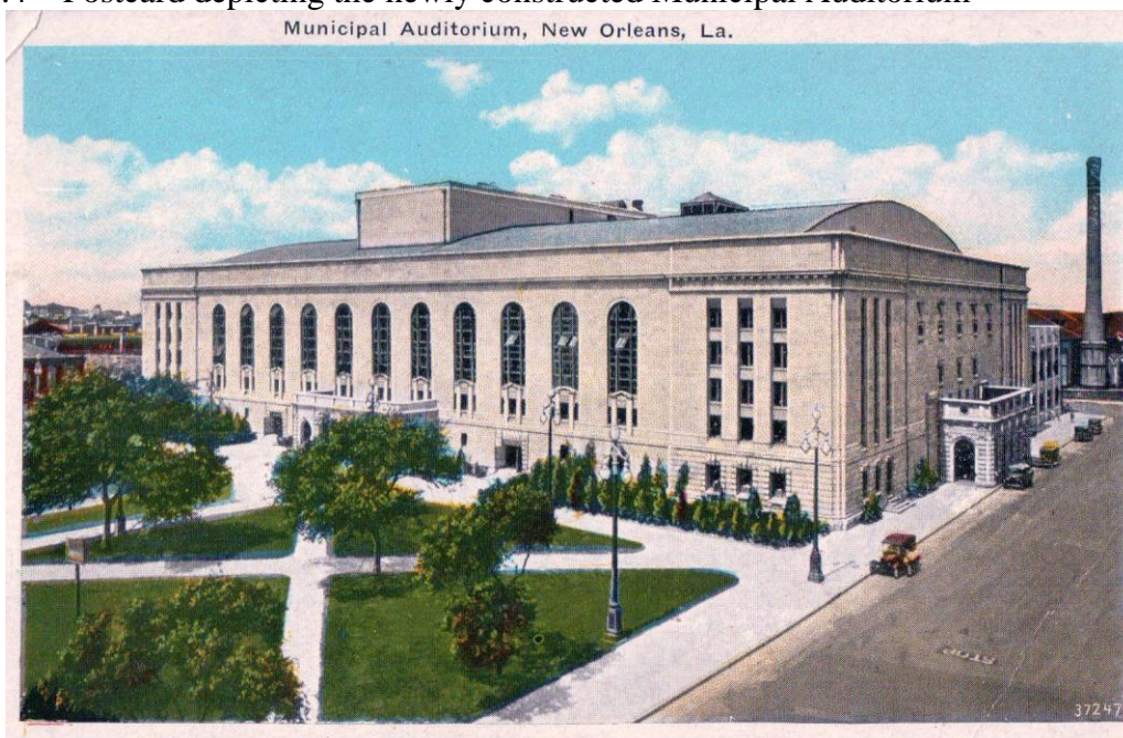
Figure 2.4 – Postcard depicting the newly constructed Municipal Auditorium 80
