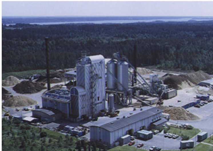
Figure 1.7 Värnamo demonstration plant (Stahl, et. al, 2004.)
