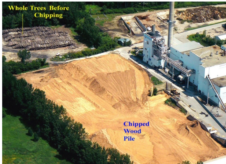
Figure 1.9 McNeil Power Station, Burlington, Vermont
