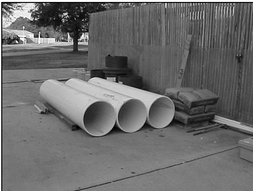
Picture 4 – Lysimeters Prior to Assembly at Pilot Plant
