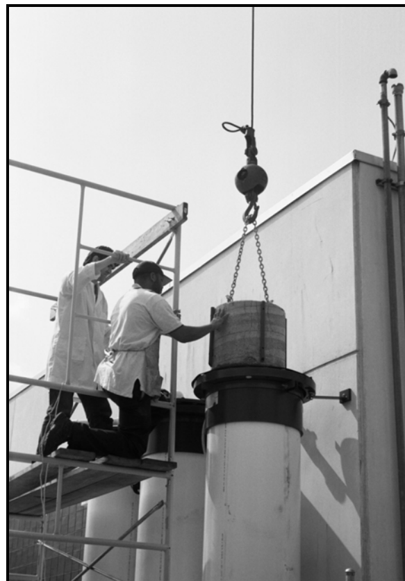
Picture 16 – Placing Concrete Weight in a Lysimeter
