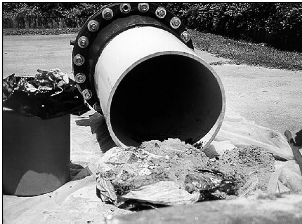
Picture 3 – Unloading Test Chamber
