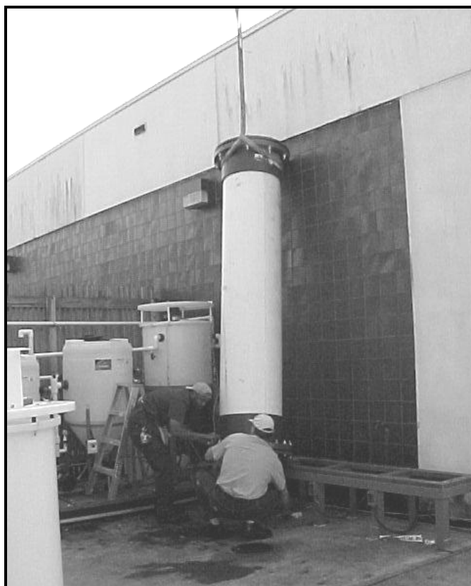
Picture 6 – Placing Lysimeter at Final Position
