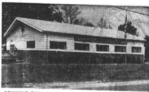
COLUMNS ELIMINATED — Truss construction is one of the features of this building recently constructed for Glen Cove Features Post 261 of Piscataway Township by American Builders of Green Brook Township. This specialized use of truss construction eliminates space-wasting columns and posts allowing for more attractive design and unobstructed floor space.
