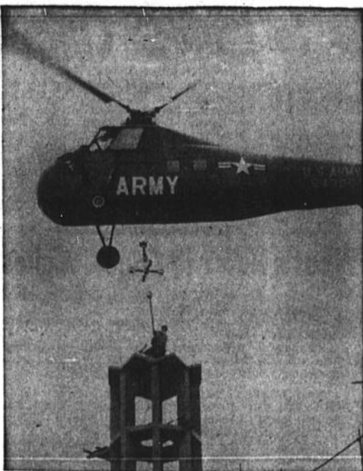
ON TARGET — On target with a cross for the spire of a new Catholic church in Pievebelvicino, Italy, is a U. S. Army helicopter attached to the 110th Aviation Company, stationed in nearby Vicenza. The six-foot cross was placed atop the 80-foot high steeple despite gusty winds and driving rain. Hundreds of spectators from the surrounding area watched and applauded the successful training operation.
