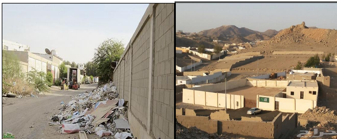
Figure 4.5: Poor Conditions in Mraykh (Source: Okaz)
