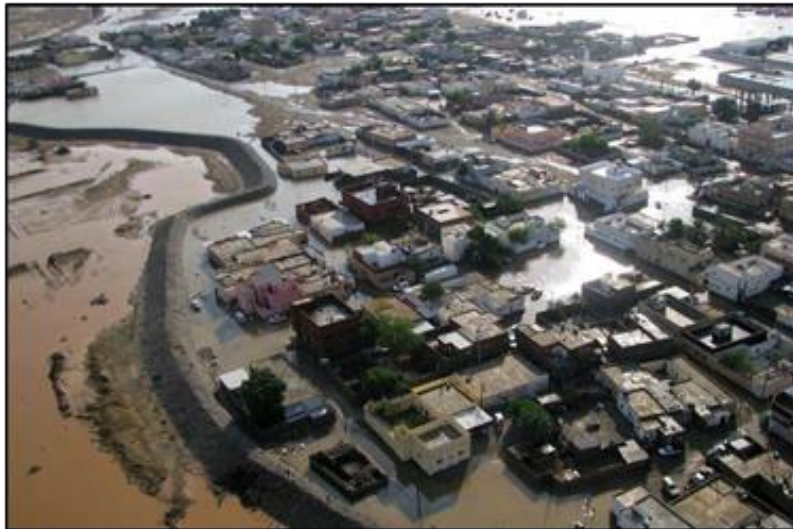
Figure 3.13: Photo of the 2009 Flooding in Jeddah (Civil Defense, 2010)
