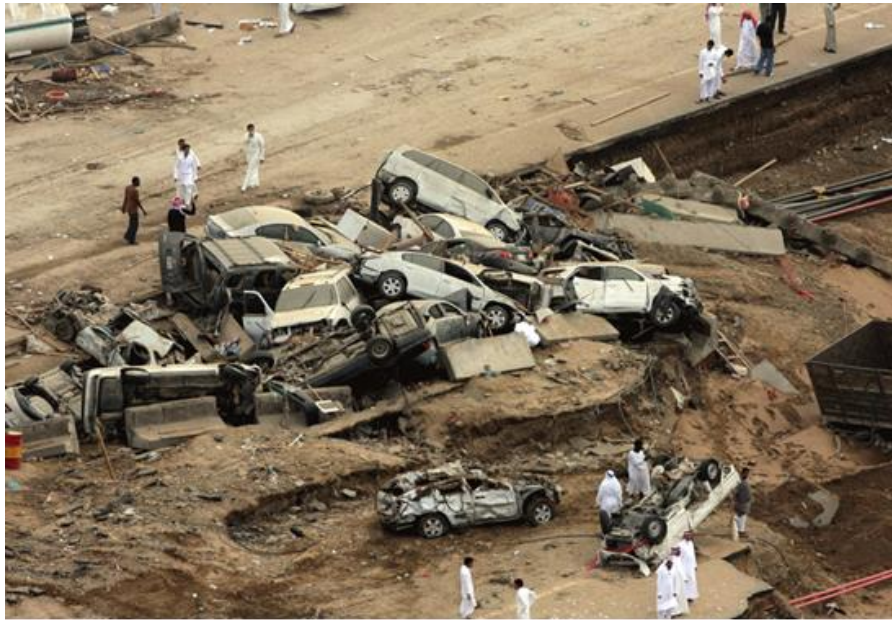
Figure 4.9: Massive property destruction in the Goyzah District (Civil Defense, 2011)
