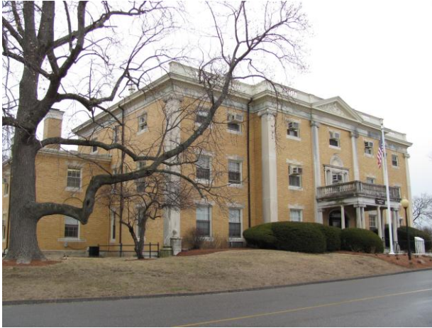
12 McLean Hospital – Administration Building
