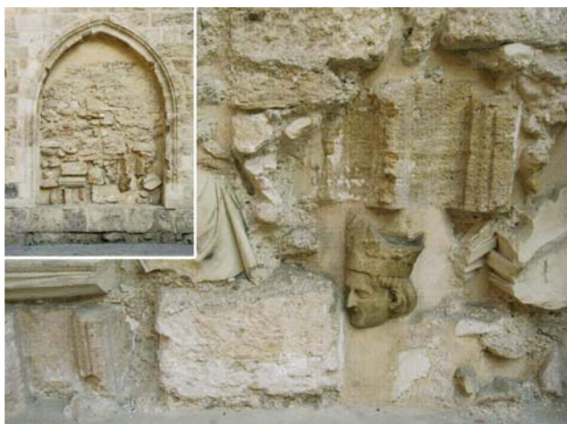
Fig. 2 Church of Santa Catalina in Valencia, Spain. Old stones, fragments and decorations used to wall up a niche of the facade
