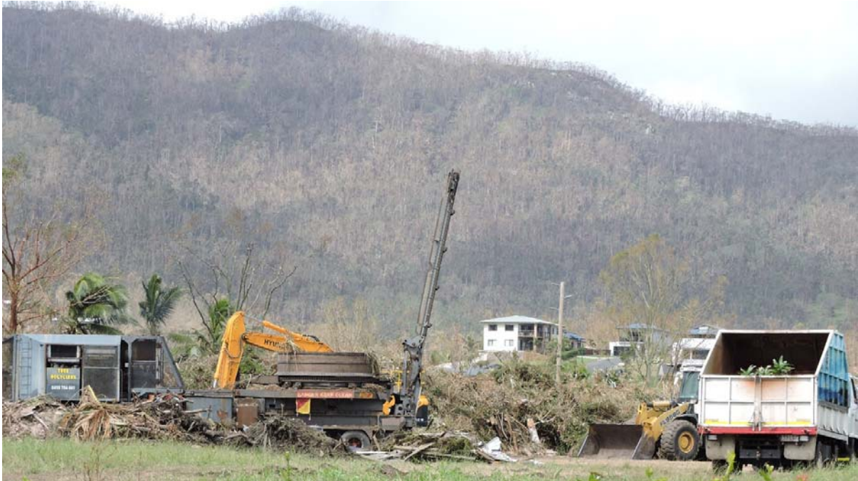
Figure 6. Temporary local green waste dump and mulching, Cannonvale
