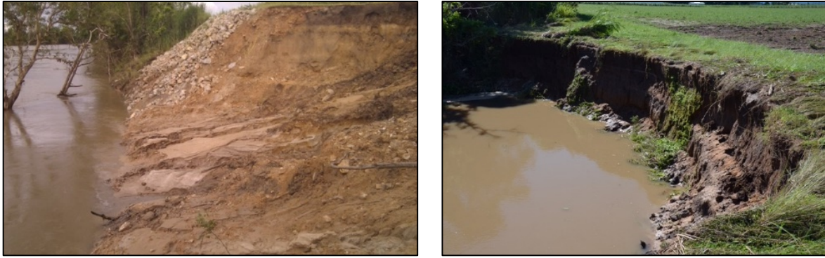
Figure 2: Landholder-supplied photos of Riverbank Erosion Reproduced with permission of landholder.
