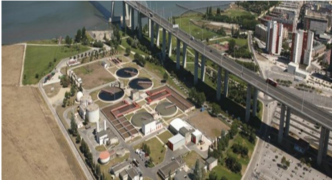
Figure 4.1 – WWTP of Beirolas
