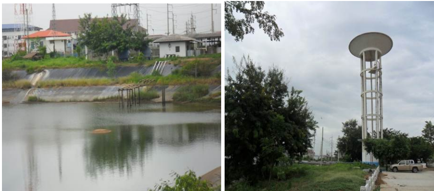
Figure 5: Picture of MSU's treatment pond and water storage
