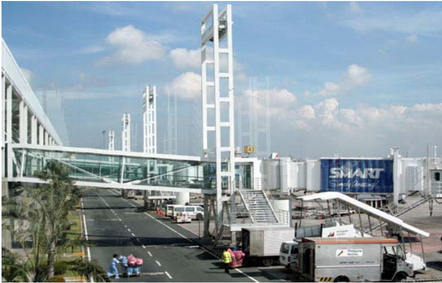
Airbridges at NAIA2 that connect the aircraft on the airside onto the landside of the airport terminal
