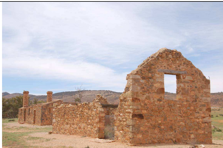
Figure 9: Abandoned Homestead Ruins Near Hawker
