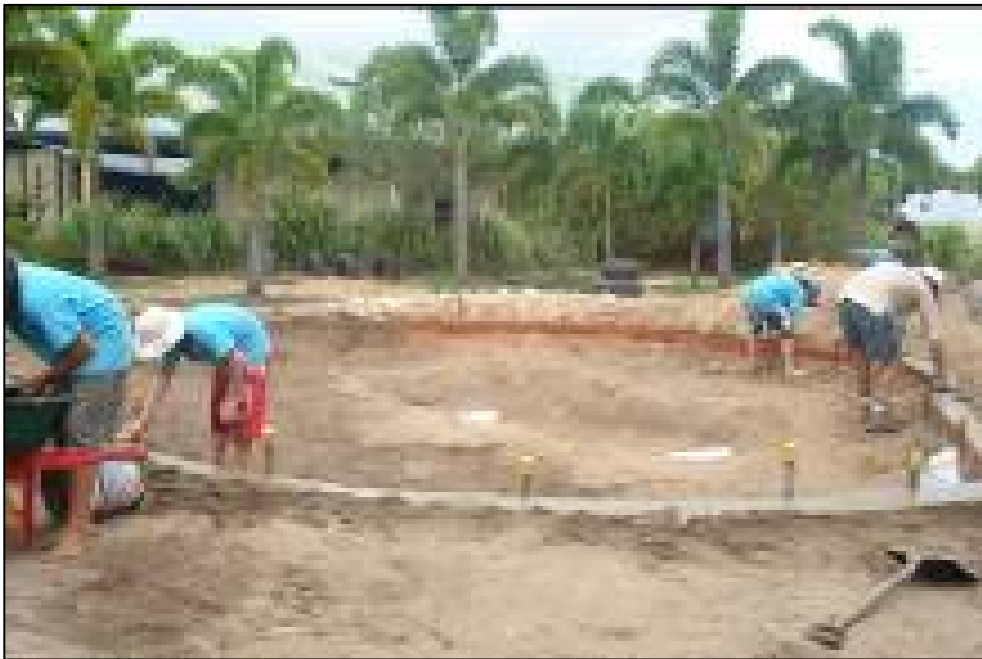
Plate 4.8. Constructing first stage of the mini wetlands at Whanilla SS
