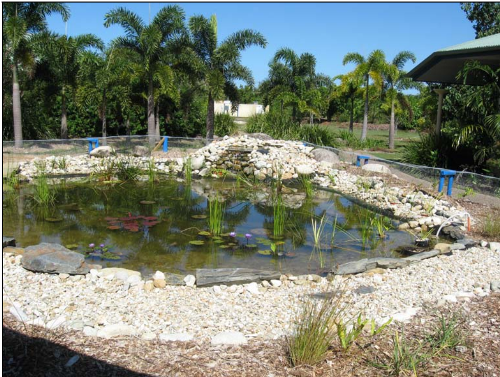
Plate 4.10. Completed mini wetlands at Whanilla SS
