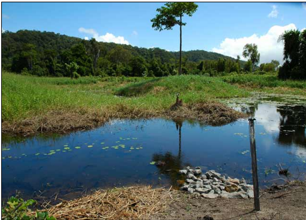
Plate 4.4. Wetlands area behind Whanilla SS after being dug out
