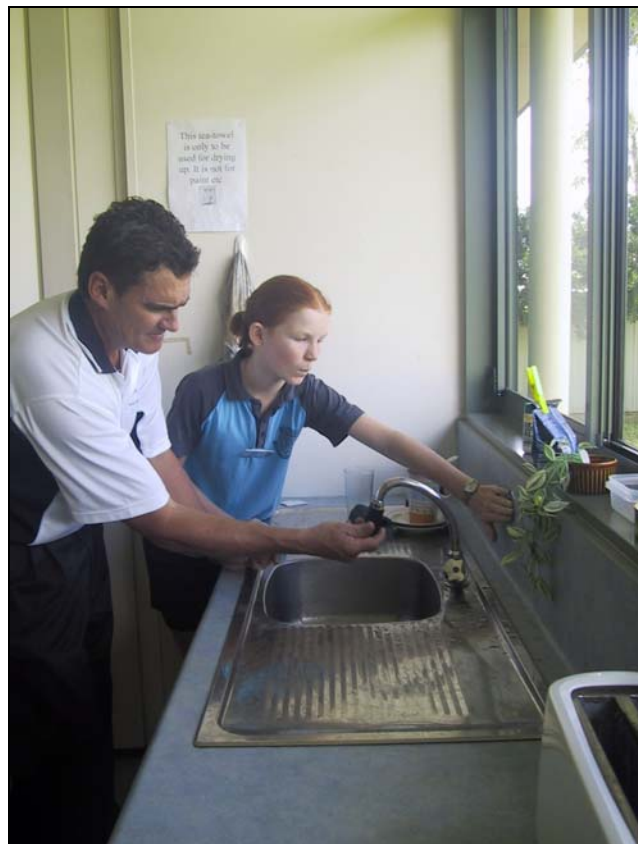
Plate 4.14. Fitting water saving devices at Hollindale SS
