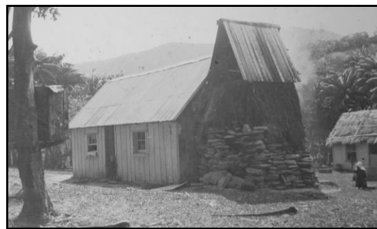
Figure 4.35: LHI Smokehouse chimney containing calcarenite blocks, palm thatch and iron. ND. Courtesy of the Lord Howe Island Museum.
