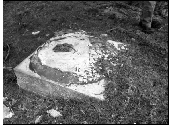
Figure 4.64: Cement tank stand with traces of cement lined iron tank that once sat on top of it
