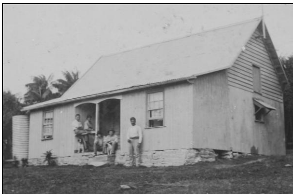
Figure 5.65: Late 19 th century LHI house with support piers cut from local calcarenite. ND. Courtesy of the Lord Howe Island Museum
