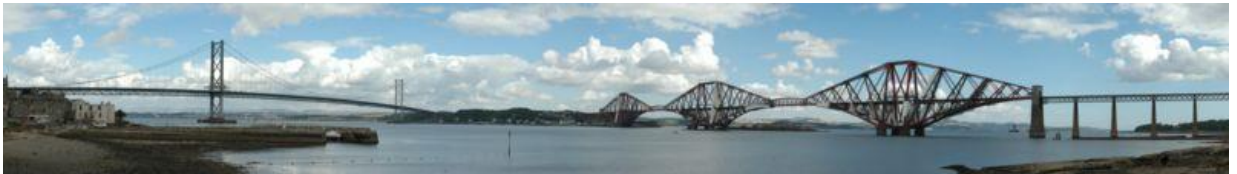
Forth Rail Bridge, Scotland (Photo: Greg Barbier - distributed via the GNU Free Documentation License)
