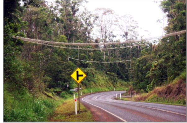
More complex rope canopy bridges erected on the Atherton Tablelands.
