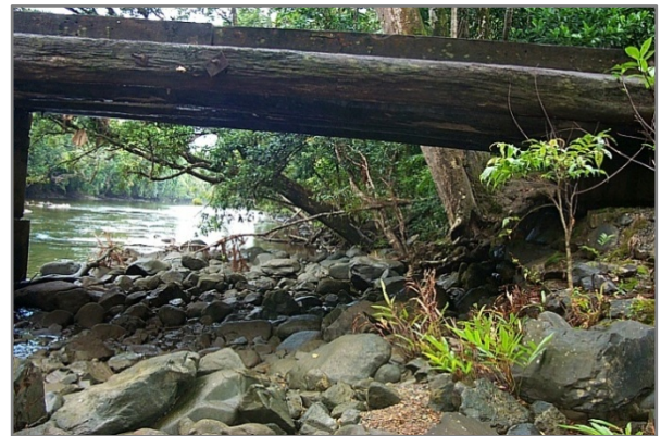
Existing bridges can, in some cases, maintain riparian habitat connectivity.
