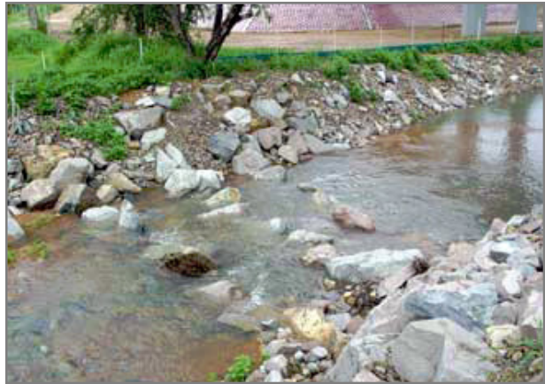
Partial width rock ramp fishway on University Creek, Townsville (Photo: Ross Kapitzke).
