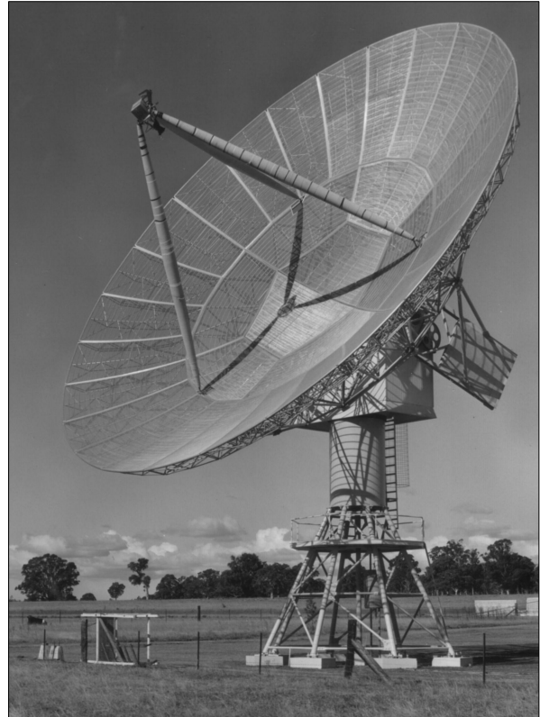
Figure 42: The 18m Kennedy Dish (courtesy ATNF Historic Photographic Archive: B6499-7).
