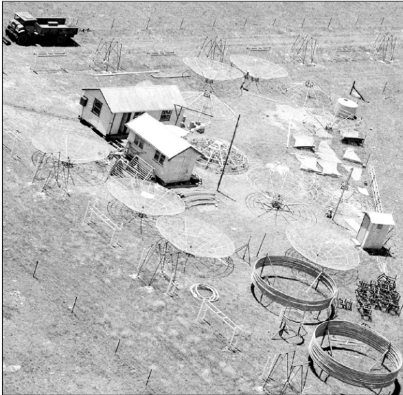
Figure 13: Aerial view showing huts, cylindrical frames and the antenna assembly area of the new Chris Cross, located very close to the central point of the Cross (courtesy ATNF Historic Photographic Archive: B5042-2).
