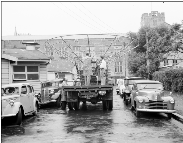
Figure 8: Loading the Chris Cross test antenna onto a truck at the RP Workshop, ready for its transfer to Potts Hill field station (courtesy ATNF Historic Photographic Archive: B3858-3).
