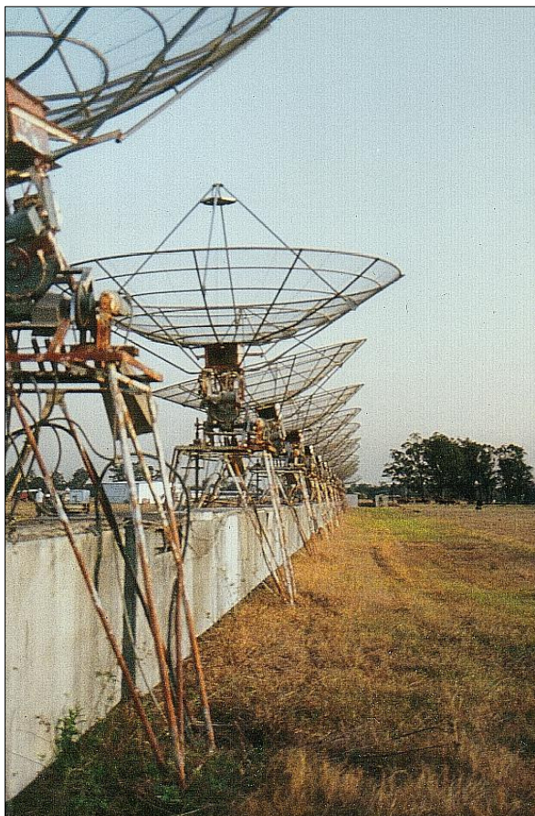
Figure 49: A view looking south along the N-S arm of the decommissioned Chris Cross showing rusting antennas (courtesy John Leahy).
