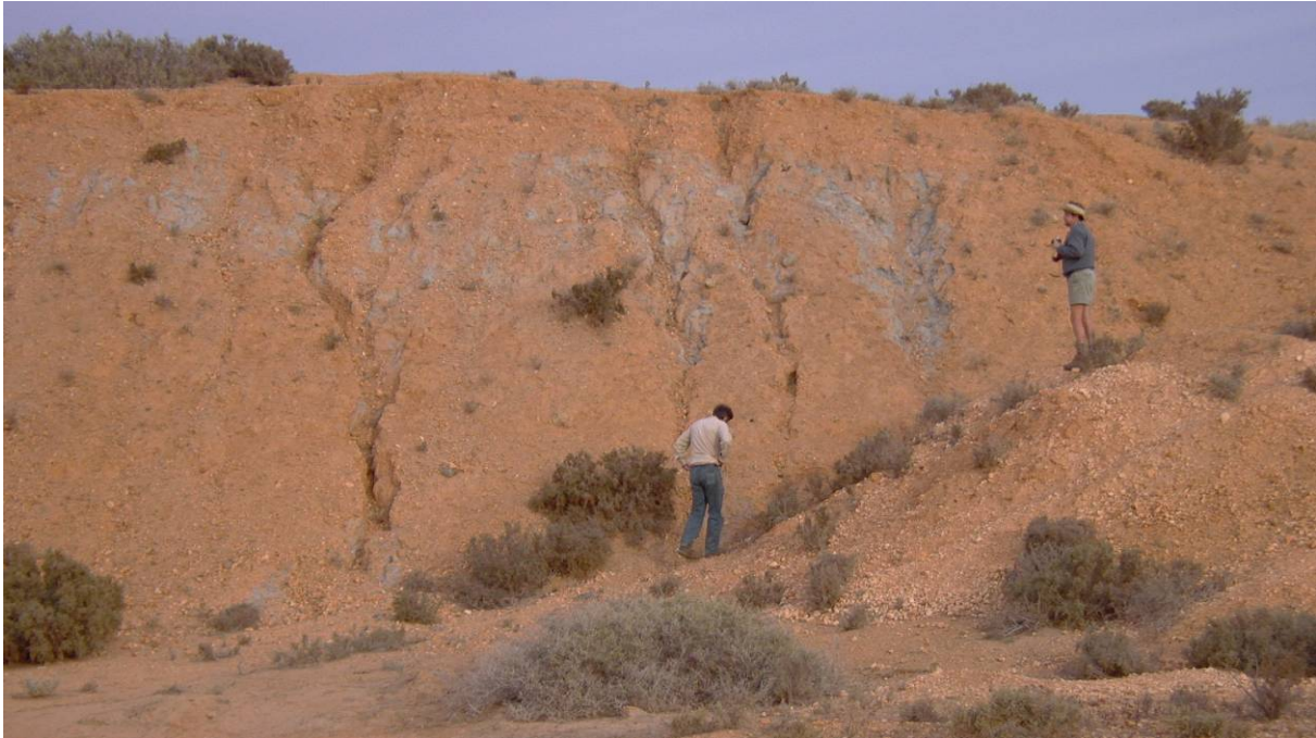
Figure 3: Rill erosion of the soil capped tailings storage facility, Radium Hill, South Australia (height of facility approximately 6 m). The soil capping is being removed, resulting in the exposure of radioactive tailings in rills.
