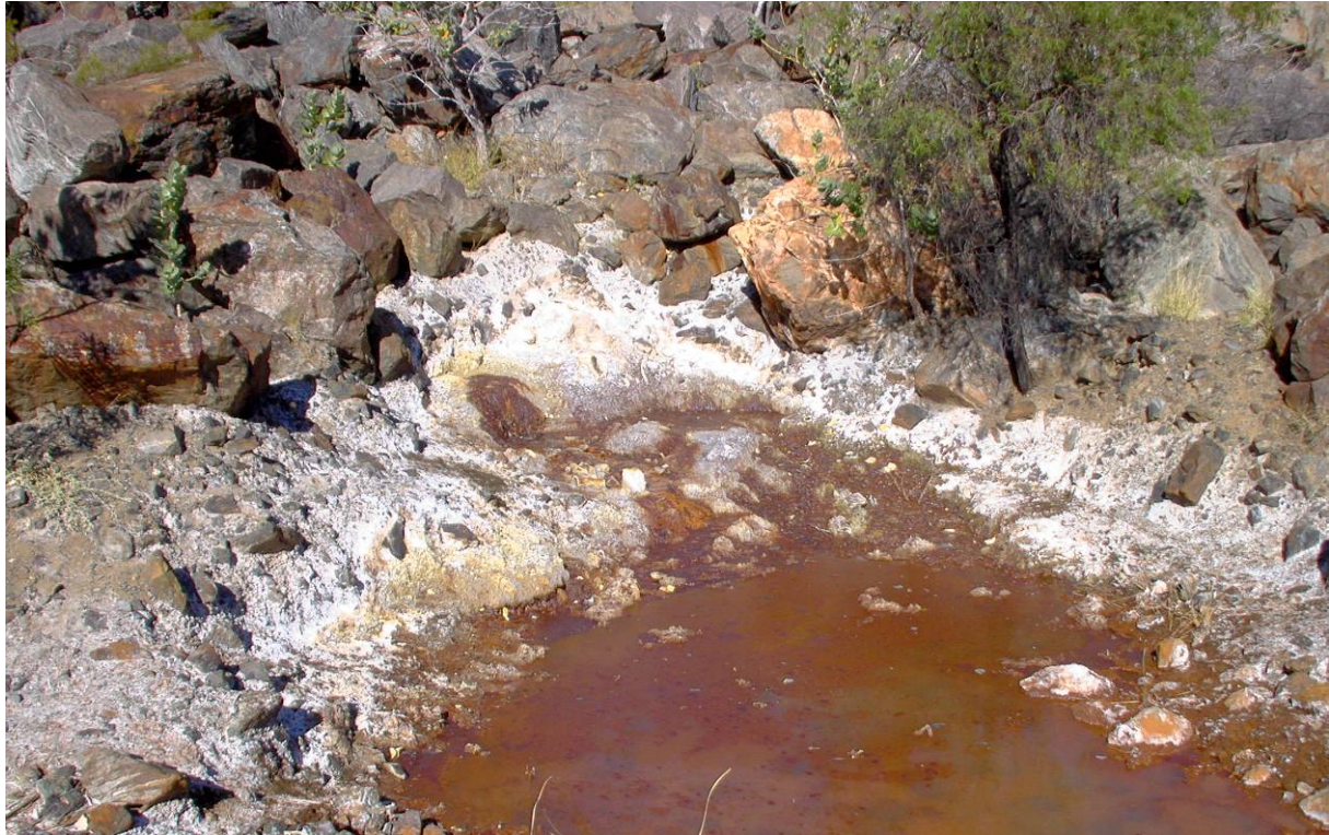
Figure 2: Seepage point at the base of the tailings dam wall, Mary Kathleen, Australia. Abundant sulfate efflorescences and Fe-oxyhydroxide precipitates form from the acid, saline, radioactive seepage water (pH: 5.5; salinity: 0.31 %). Boulders in the retaining wall are approximately 1 m in diameter.
