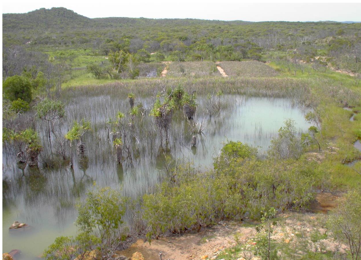
Figure 5: Wetland at the Horn Island gold mine, Australia. The wetland has failed because an adjacent damwall was constructed using acid generating waste rocks (foreground), which resulted in significant ARD and caused plant death.
