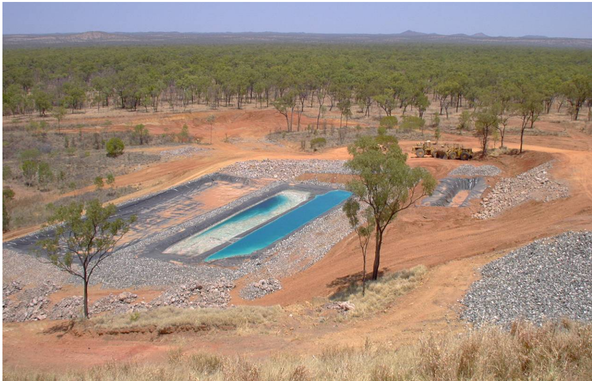
Figure 4: View from the tailings storage facility, Red Dome gold mine, Queensland, Australia. Cyanide-bearing seepage waters (~200-500 mg/l total cyanide, 80-300 mg/l WAD cyanide, 200-600 mg/l Cu) emanate from the capped tailings repository. The seepage is collected via a series of ponds where chemical degradation of cyanide and precipitation of copper cyanide salts occur. The passively treated effluent is discharged to the local stream system.
