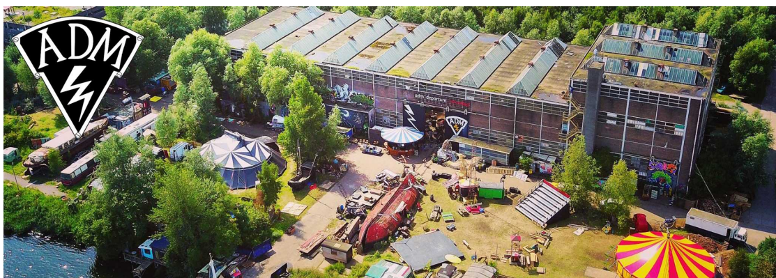
Drone image of ADM's main workshop facilities, the circus tent and various other installations and stages for performances (source: ADM).
