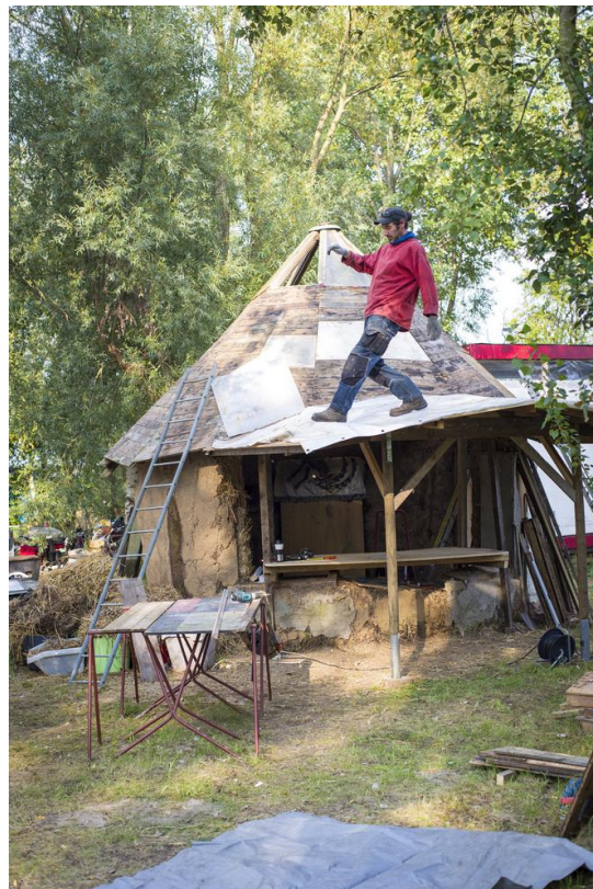
An ADM dwelling made out of cob, natural building and recycling of disposed materials for the creation of houses, art and objects of craft are typical practices in ADM (source: ADM)
