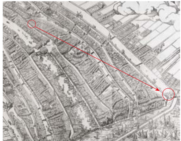
29 Detail of fig. 27. The red circle on the left marks the workshop of Jacob Cornelisz van Oostsanen, the one on the right the Haarlemmerpoort
