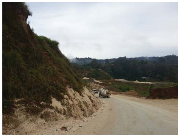
Figure 4. Spine Road to Wellpads, PNG LNG Project, Hides.
