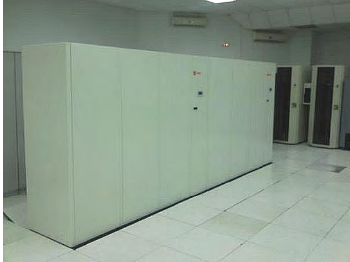
Figure 6: Air-conditioning cabins.
