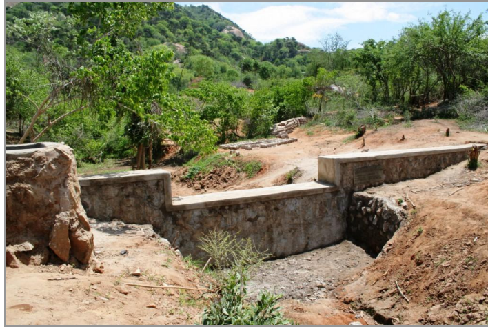
Figure 1.3 A new build dam without any sand accumulated behind it yet. The spillway is in the middle of the dam.
