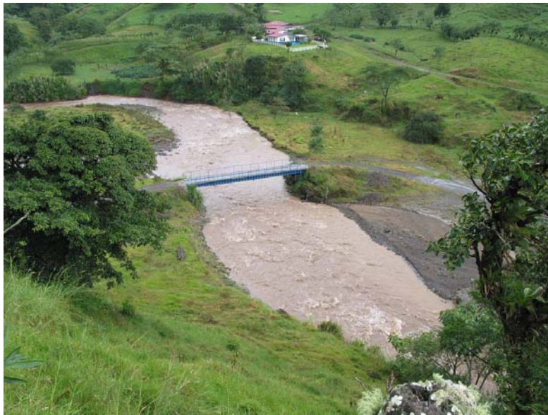
Figure V.3. Example of a natural channel section with a constriction afforded by a bridge (Lower Rio Chiquito, northern Costa Rica).
