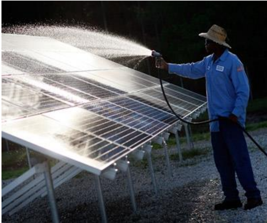
Figure 3.4: Dust removal using water blowing method
