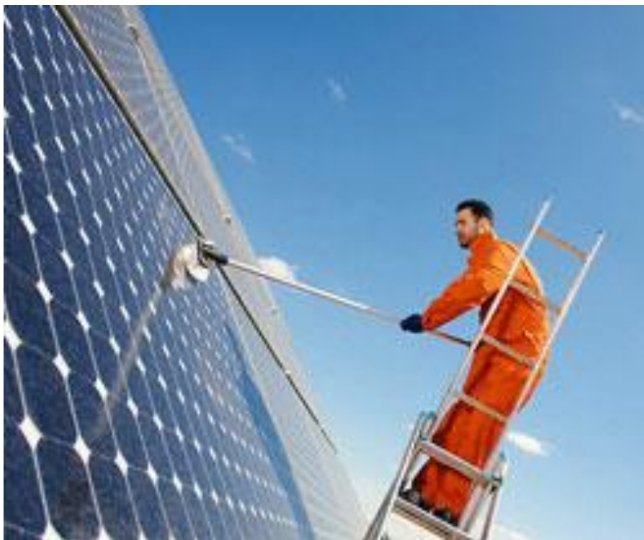
Figure 3.5: Dust removal using brush method
