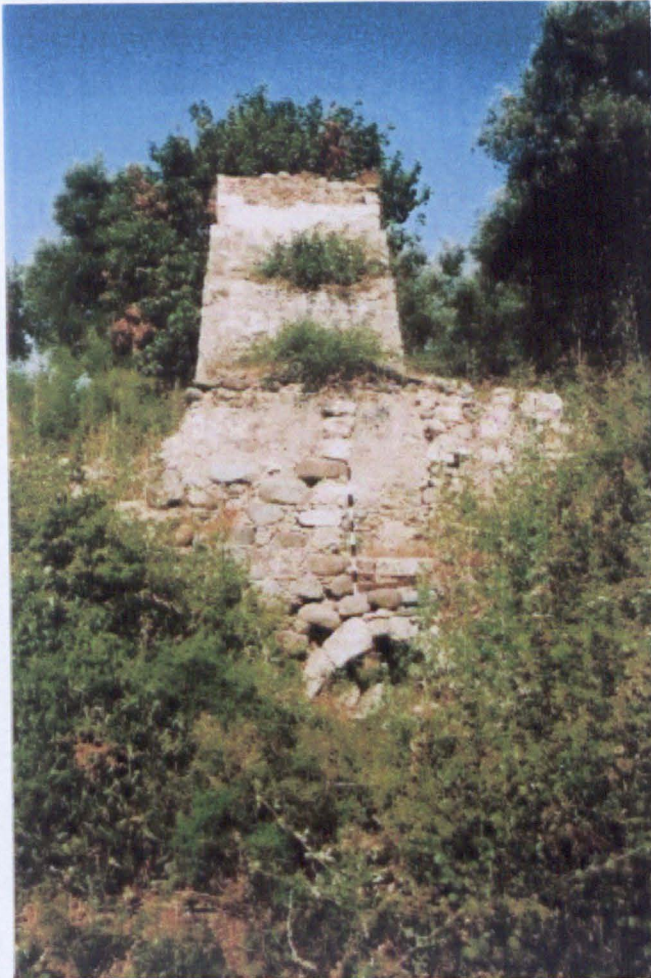
Figure 5.83. Penstock and wheel chamber, BU0044.
