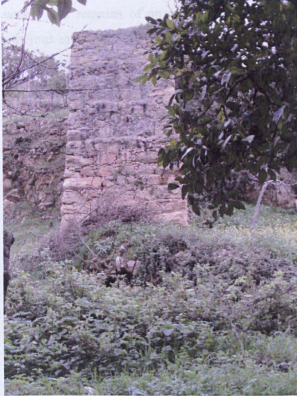
Figure 5. 18. Penstock and view of entry to wheel chamber, RJB2.
