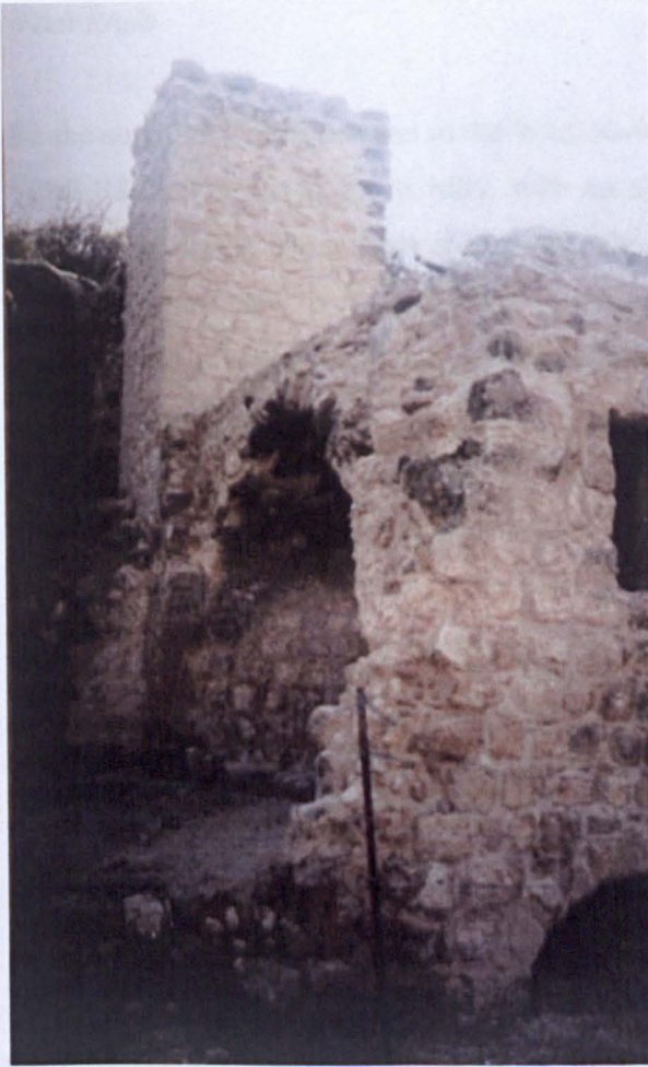
Figure 5. 15. Restored penstock and remains of mill house, Wādi Rayyān. Courtesy of Dr. Rami Daher, Jordan University of Science and Technology.
