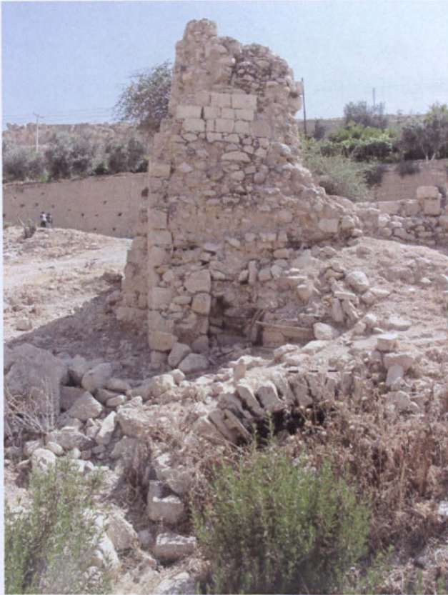
Figure 5. 53. Penstock and arched entrance to wheel chamber, with in situ millstones above, SK3.
