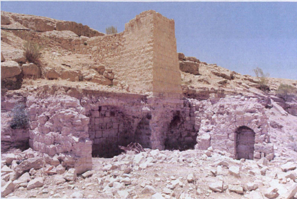
Figure 5. 42. Penstock and remains of mill house with blocked entrance.
