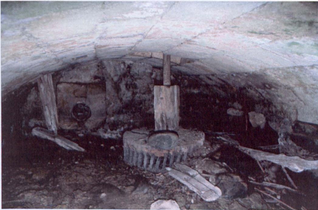
Figure 5. 88. Inside of wheel chamber, BU0070. Remains of wooden paddles which were once attached to the wheel are scattered around the chamber. (Photo: Chris Parks)
