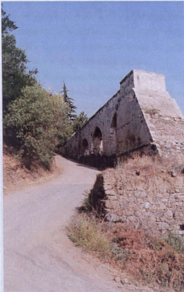
Figure 5. 86. Triple-arched millrace and penstock, with remains of mill house in the foreground, BU0075.
