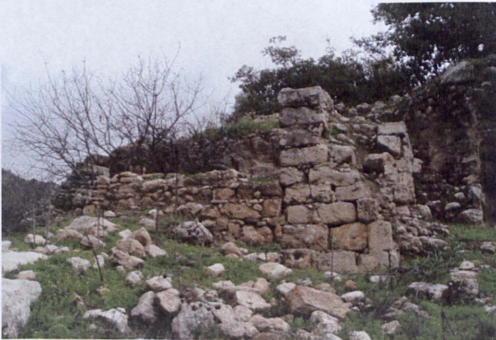
Figure 5. 17. Remains of penstock and mill house, RJB1.
