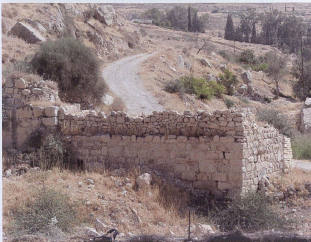
Figure 5. 55. Remains of penstock, mill house and wheel chamber, SK4.
