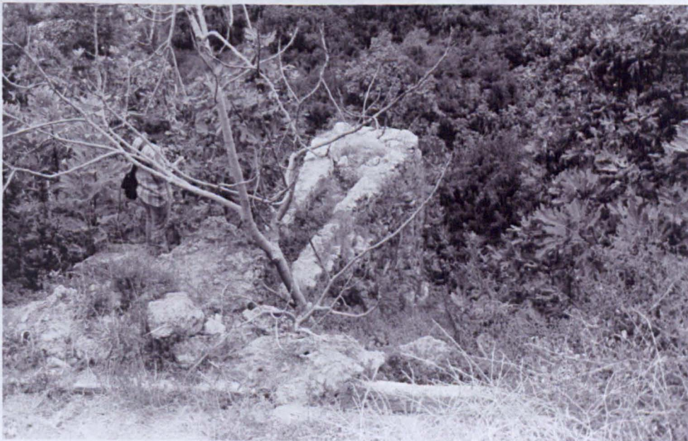
Figure 5. 11. RAY3, view of penstock from above; the modern concrete channel runs perpendicular to it.
