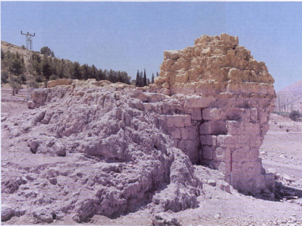
Figure 5. 40. Remains of penstock and collapsed millrace, WĀL3.
