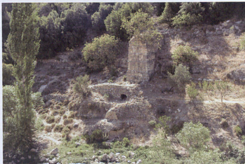
Figure 5. 4. View of penstock and remains of wheel chamber, KFR.
