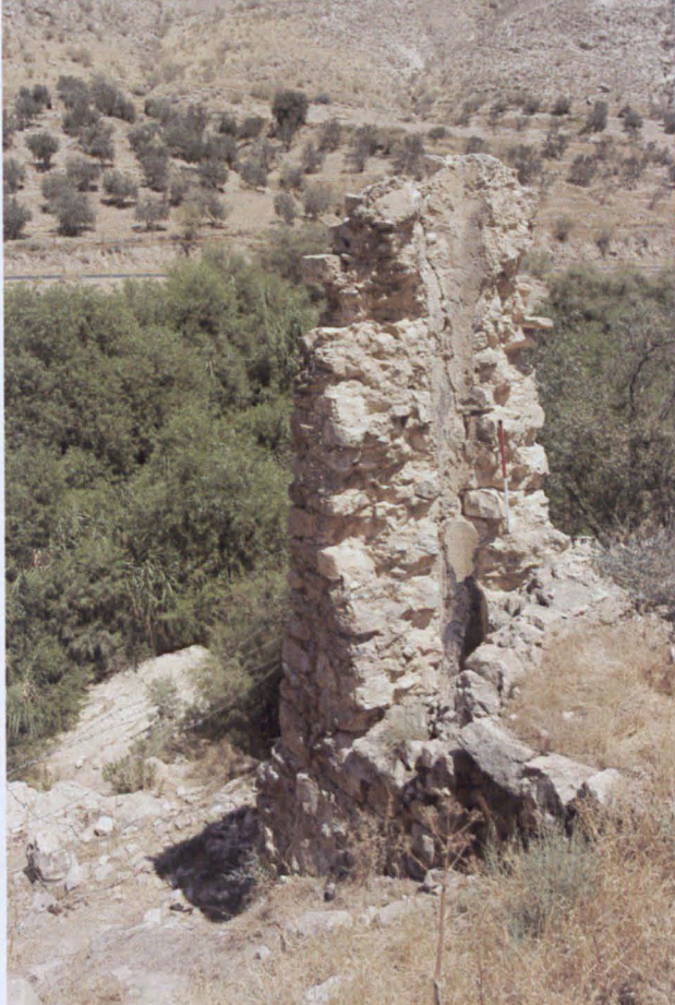
Figure 5. 44. Remains of penstock and plaster lined chute, WH7.
