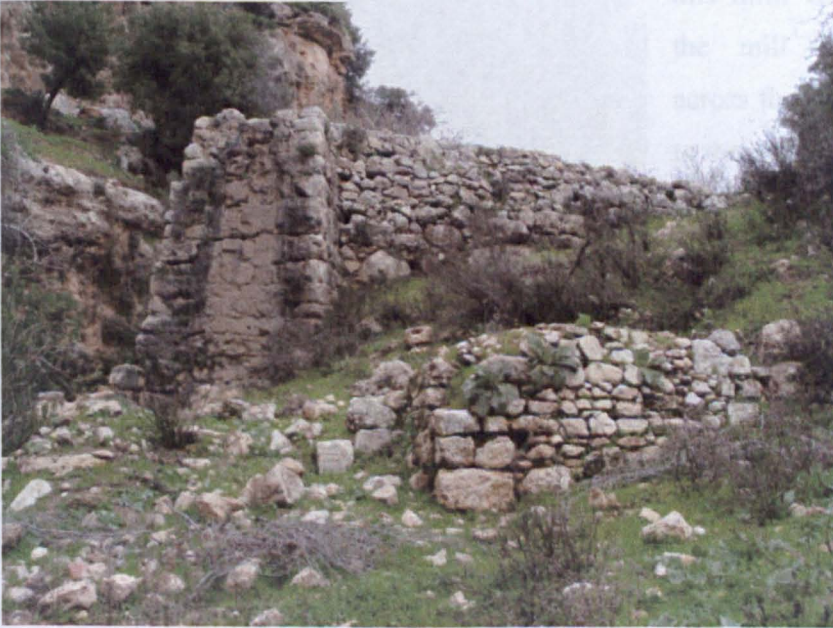
Figure 5. 19. Remains of penstock and possible mill house, RJB3.
