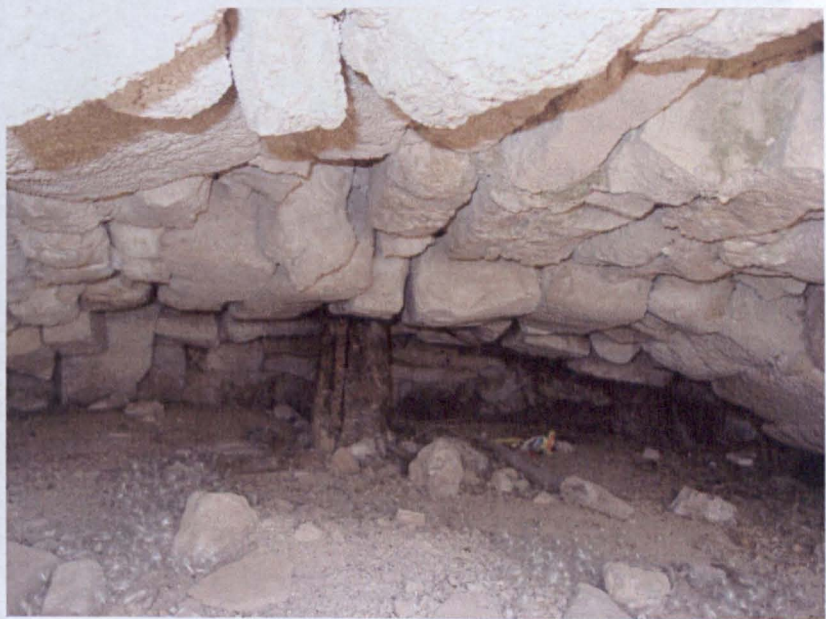
Figure 5. 54. Inside wheel chamber; the wooden shaft connecting the wheel to the millstones above is still in situ.
