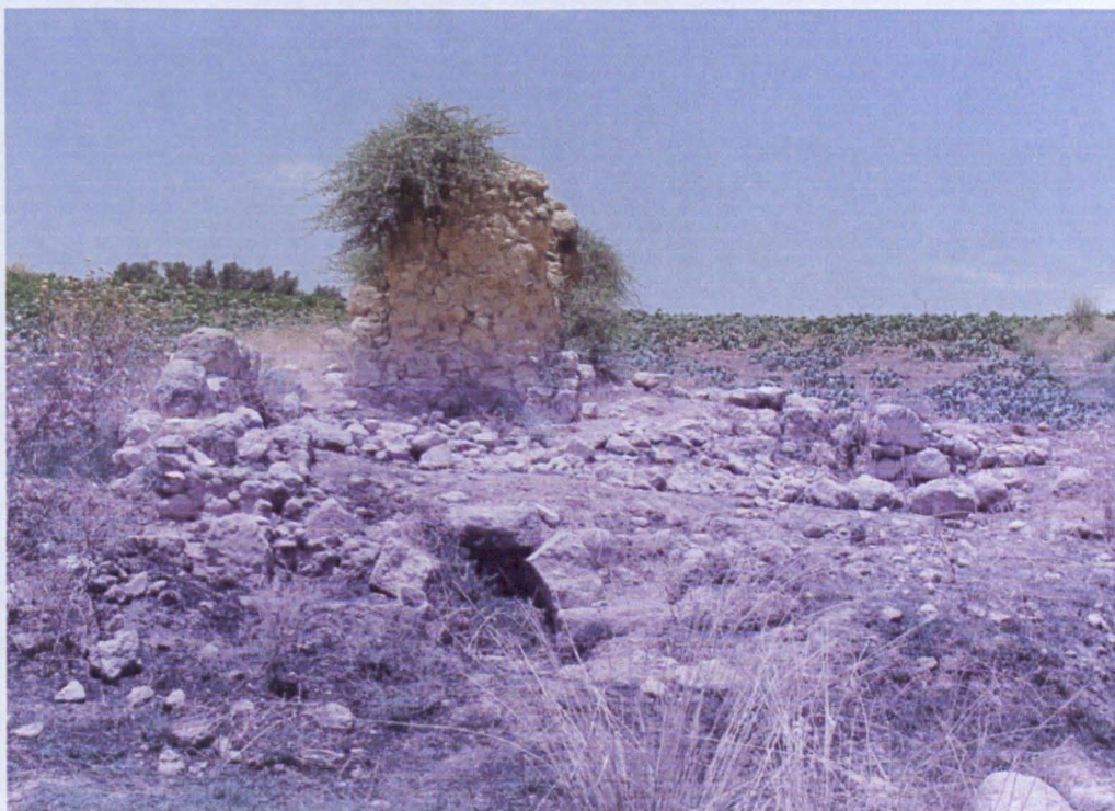
Figure 5. 33. Remains of penstock and collapsed mill house, with arched opening to wheel chamber visible below.
