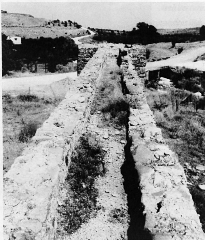
Figure 5. 94. View of millrace and penstock chute, BU0073.
