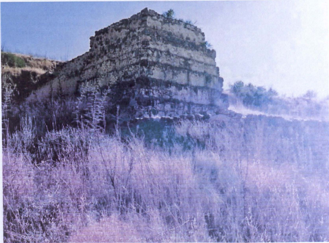
Figure 5. 97. Penstock and remains of mill house, BU0096.
