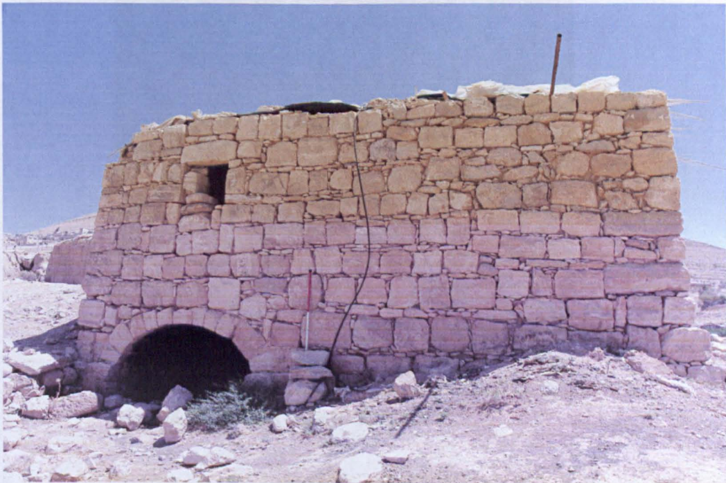
Figure 5. 38. WĀL1, entrance to wheel chamber and view of mill house.
