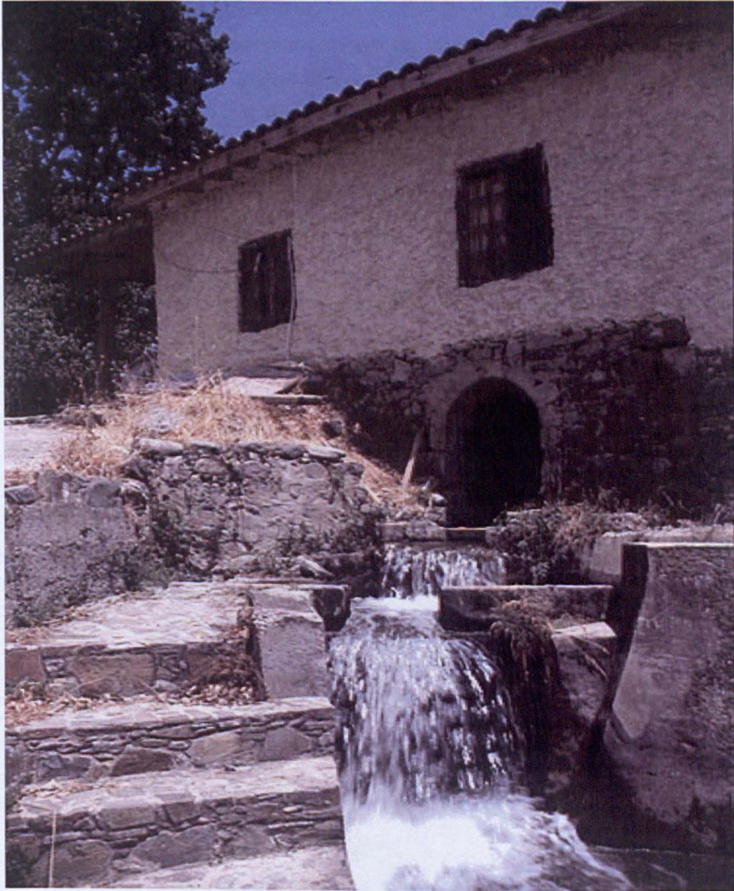
Figure 5. 91. Mill house and wheel chamber on a working day, BU0049. (Photo: Chris Parks)
