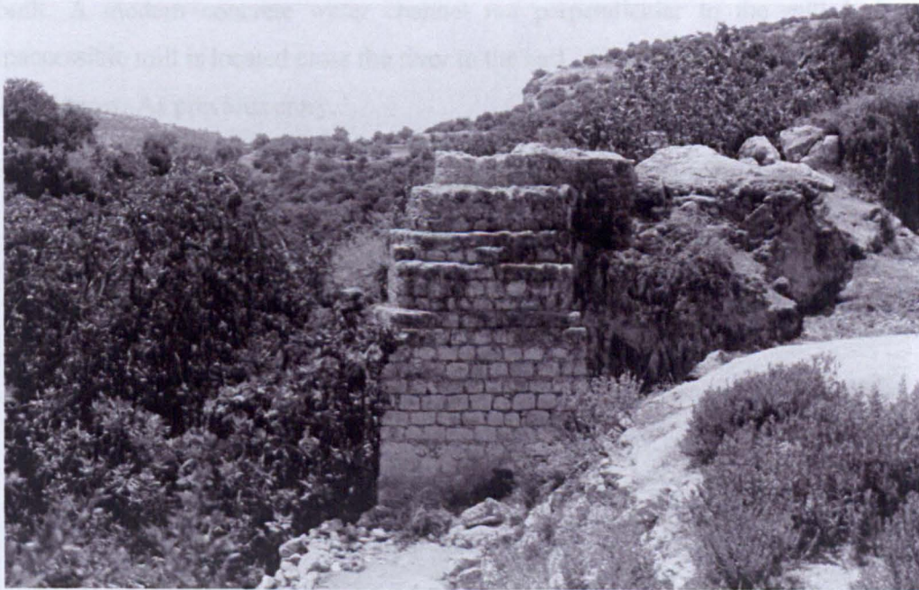
Figure 5. 10. Stepped and twisting penstock, RAY2.
