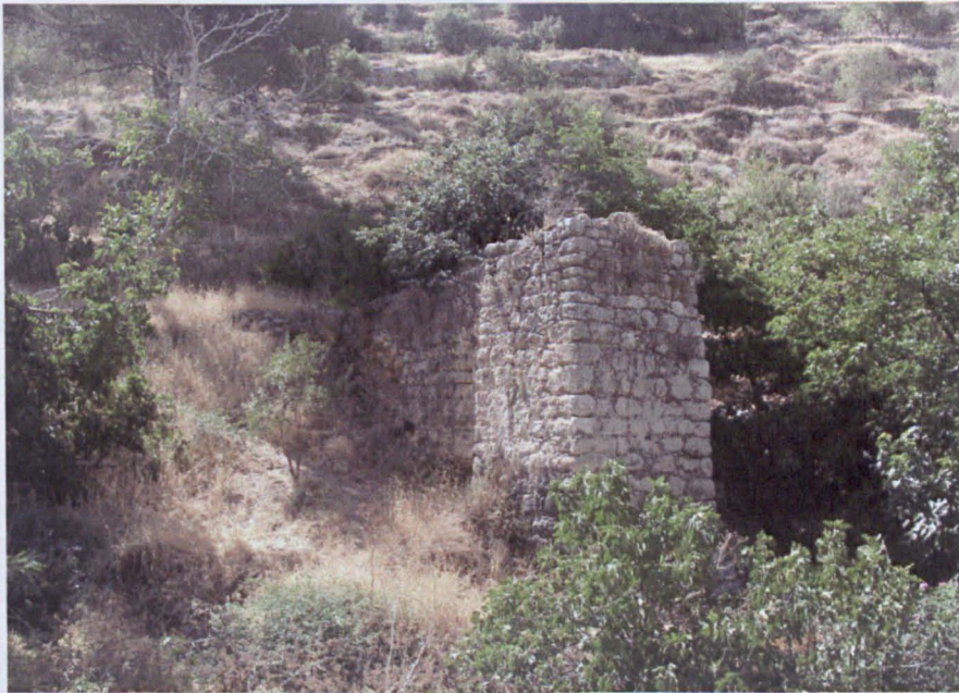
Figure 5. 22. View of penstock, SHU1.
