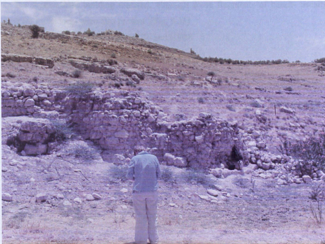
Figure 5. 34. Collapsed penstock and wheelhouse, ḤSB6.
