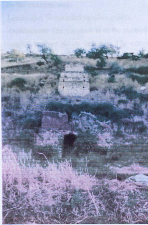
Figure 5.95. Penstock and wheel chamber, BU0104.
