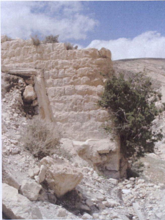
Figure 5. 59. Remains of penstock, SBK1.
