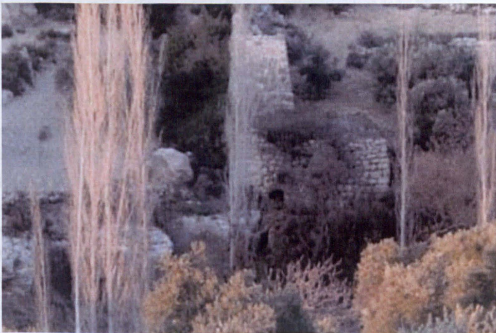
Figure 5. 7. Penstock and mill house, KFR6.; the opening to the wheel chamber can be seen directly below the arched window of the mill house.
