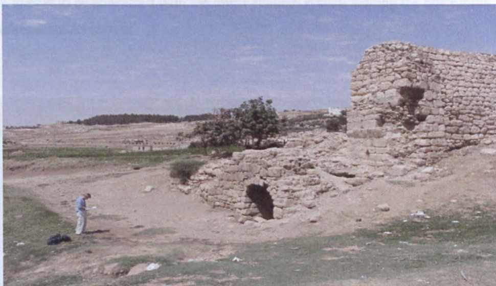
Figure 5. 29. View of penstock and collapsed wheel chamber, ḤSB1.
