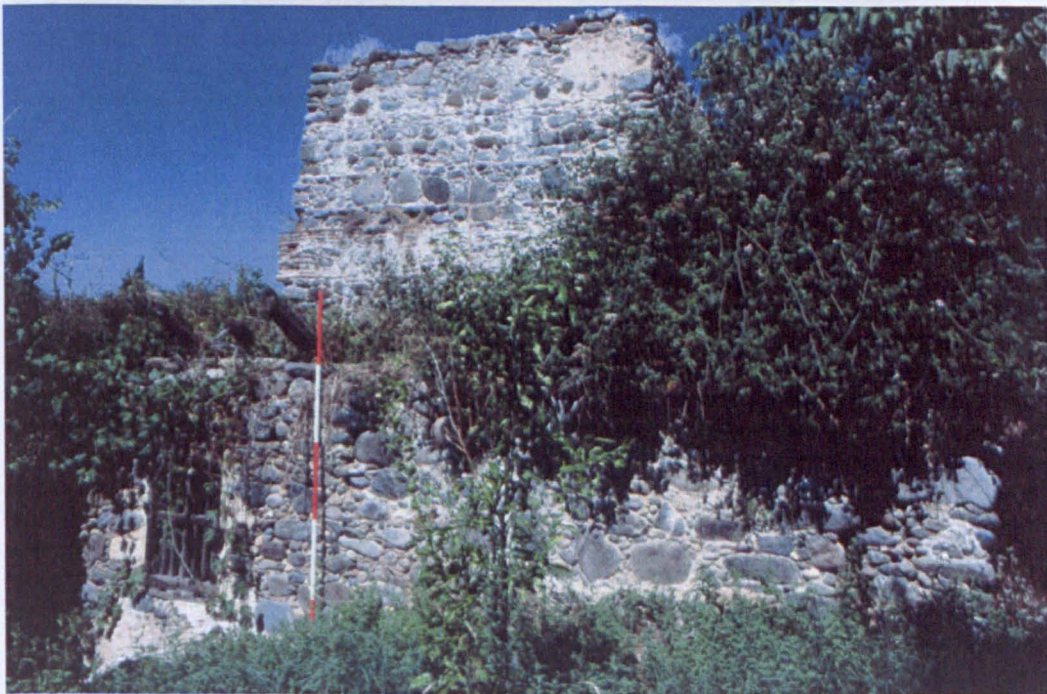
Figure 5. 87. Penstock and remains of mill house, BU0070. (Photo: Chris Parks)
