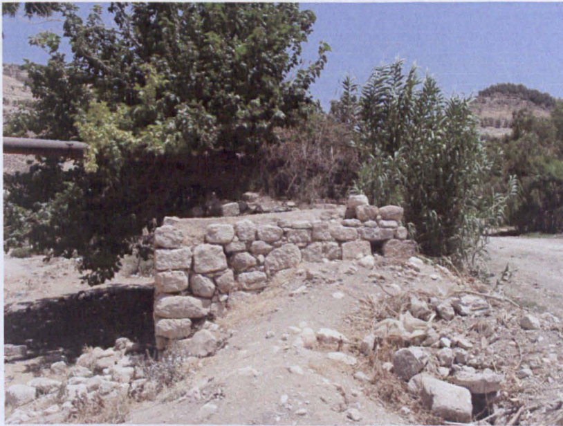
Figure 5. 50. Remains of penstock, SK1.
