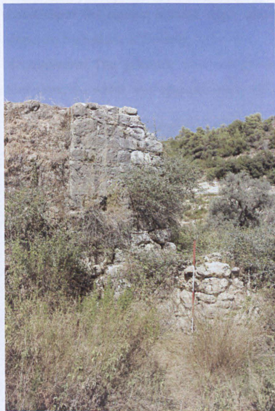
Figure 5. 3. Penstock and collapsed mill house, KFR2. (Photo: Denis Genequand)
