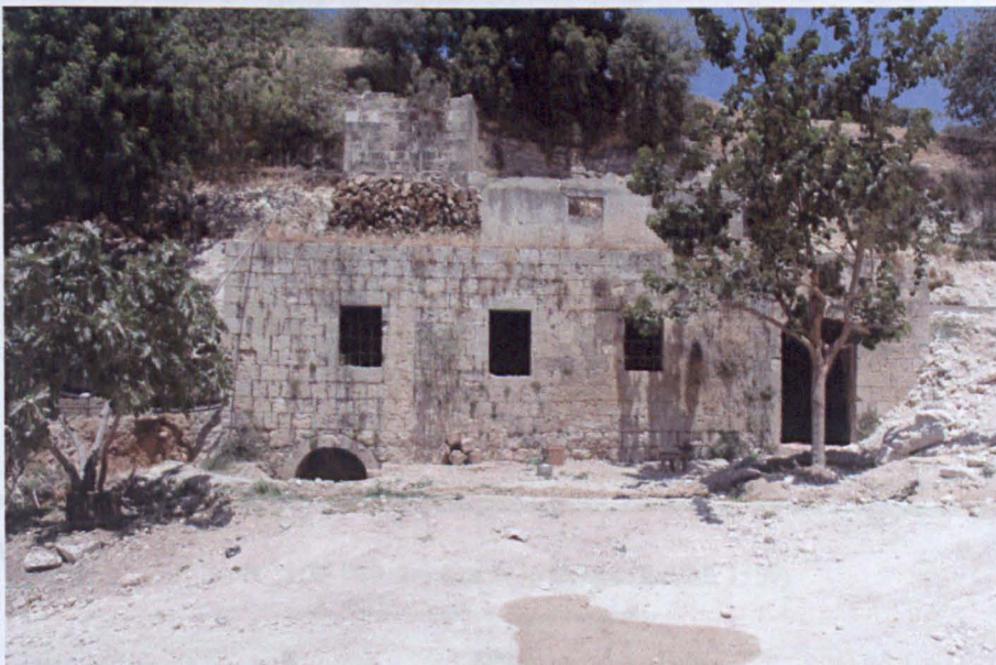
Figure 5. 27. Partially restored mill, SĪR2, Wādi al-Sīr.
