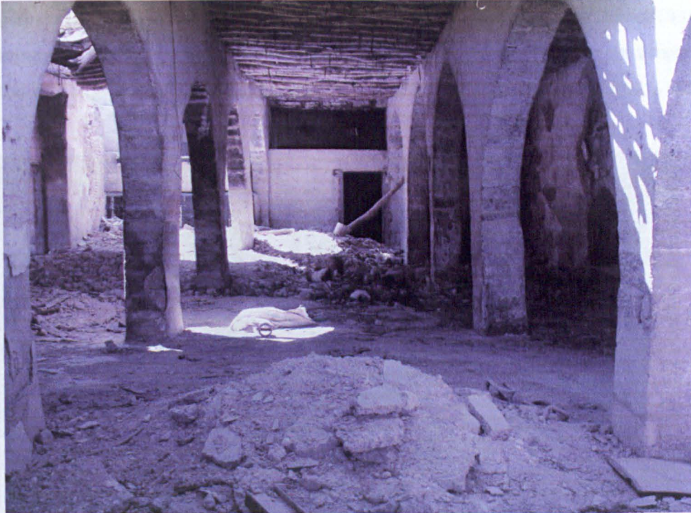
Figure 5. 70. Inside of mill rooms, DAM1.
