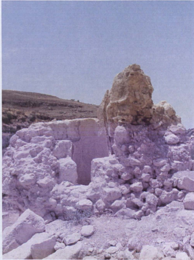
Figure 5. 36. Remains of plaster lined chute, double-penstock mill, HSB8.
