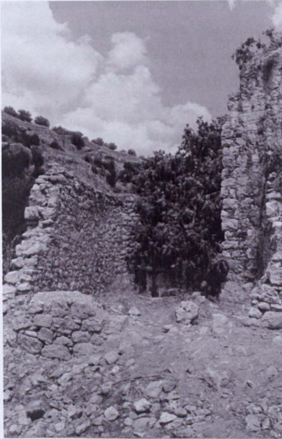
Figure 5. 9. RAY1, penstock and remains of mill house.
