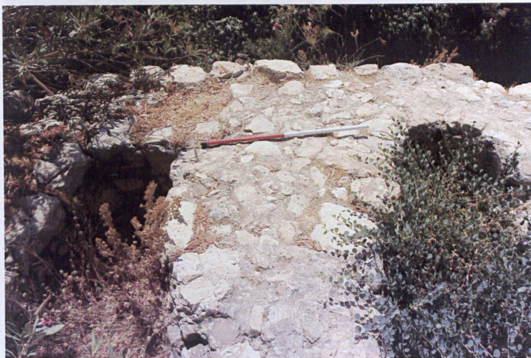
Figure 5. 43. Twin-chute penstock, WH6.
