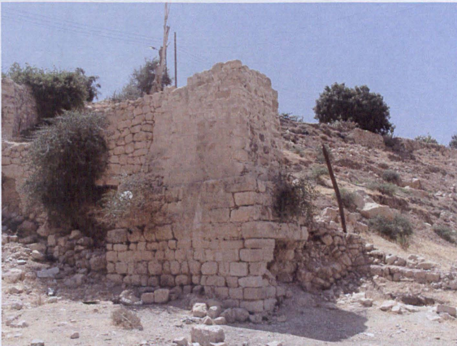
Figure 5. 51. Remains of penstock and millrace, SK2.
