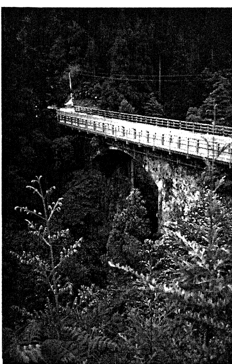
Figure 9.18: Masonry bridge
