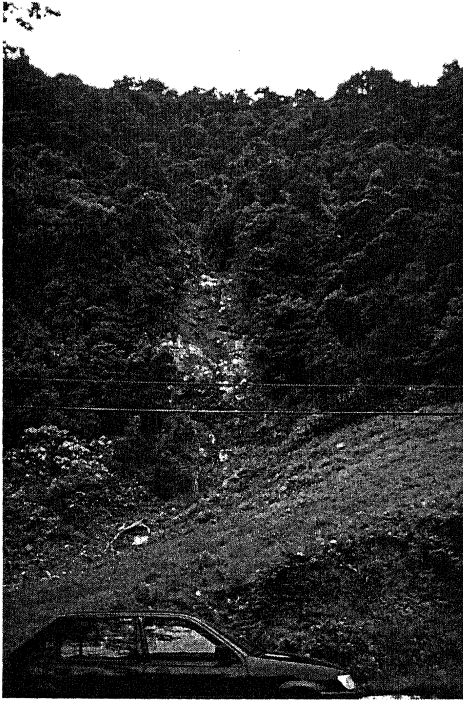
Figure 9.6: The scar left by a recent, small scale, landslide.
