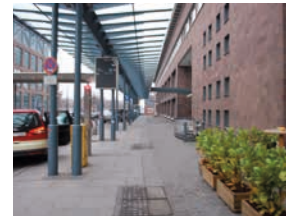
fig. 89 Bremen Airport Main Entrance
