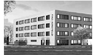
fig. 71 and 72 The ENT (Ear-Nose-Throat doctor) practice in the FAZ medical center building, Krefeld, Germany.
