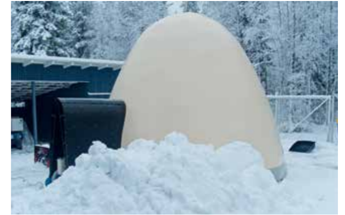
p. 6 Catenarian curve-shaped air pressure mould (RAMK 2010).
