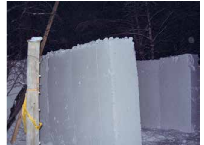
p. 1 Free-standing snow breastwork of even thickness (Ryynänen 2011).
