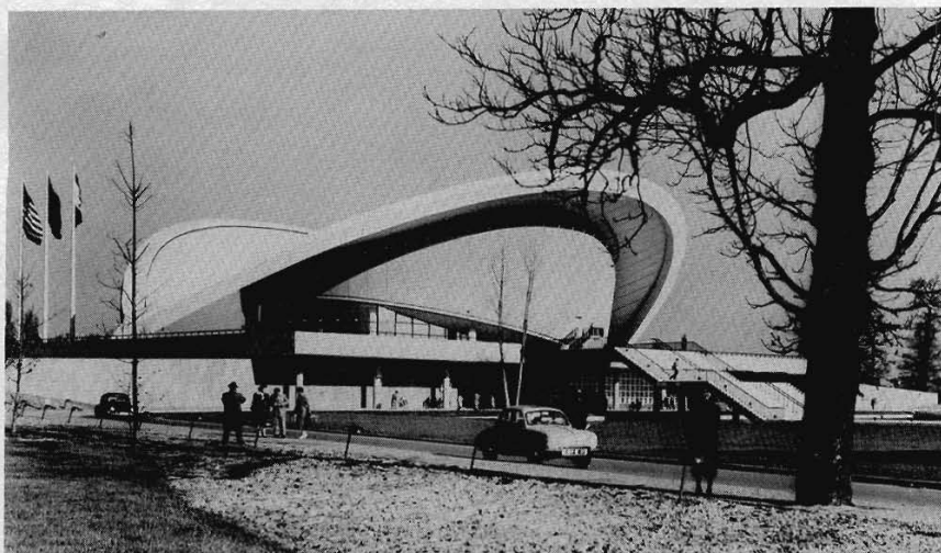
FIGURE 14. The Congress Hall as executed (courtesy of Hugh A. Stubbins and Associates, Cambridge, Mass.).
