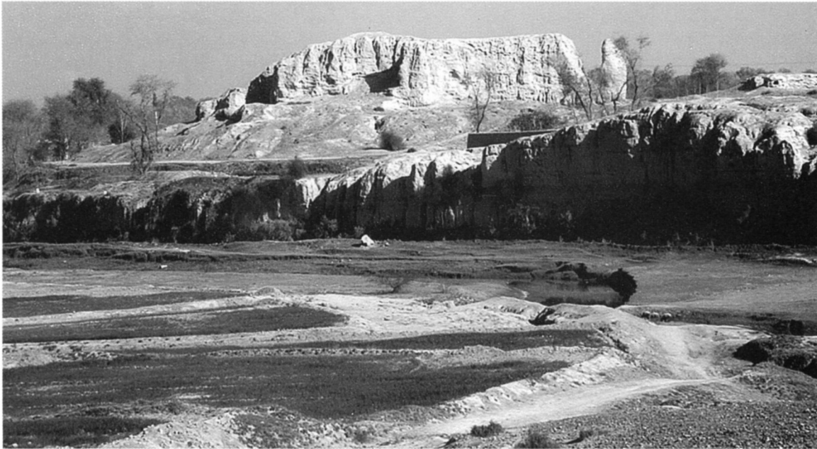
Fig. 4. View toward west of citadel in area A. Lohra nullah is in the foreground.
