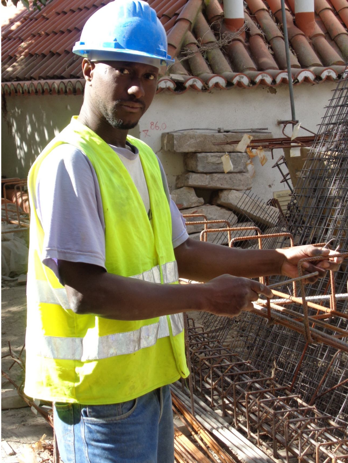
DI_L_R1 Working in a construction site (photo taken by RI/L/R1).
