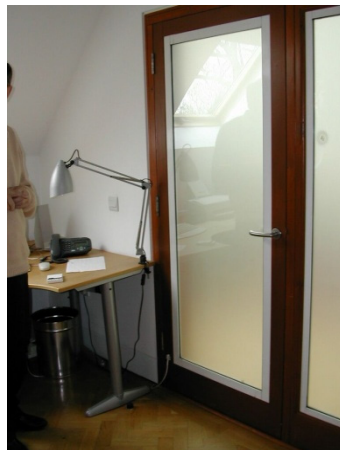
Figures 162 – Door with glass that changes from transparent to translucent at the turn of a switch. Millenium House, London (photo: SE 2003).
