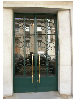
Figures 86 – Entrance doors to the building (photos: SE 2010)
