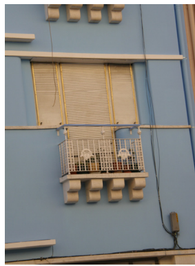
Figures 175 – telecommunications infrastructures mounted on facade. (photos: SE 2010)
