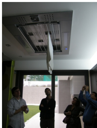
Figure 120 – Equipment for drying clothes using jets of hot air. Kasa do Futuro, Ericeira (photo: SE 2009)
