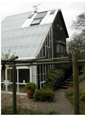
Figure 46 – Use of photovoltaic solar panels to heat domestic water and generate electricity (to supplement energy from the concessionary). Millennium House, Integer project, Watford (photo: SE 2004)
