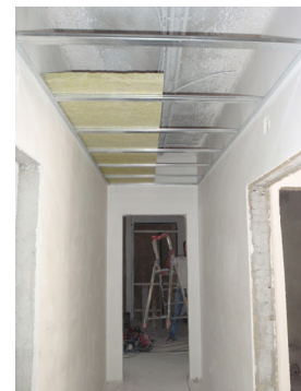
Figure 185 – Suspended ceiling in rehabilitated dwelling hiding cables (photo: AC 2008)
