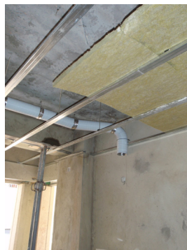
Figure 184 – Suspended ceiling in rehabilitated dwelling hiding extraction tube and beam. (photo: AC 2008)
