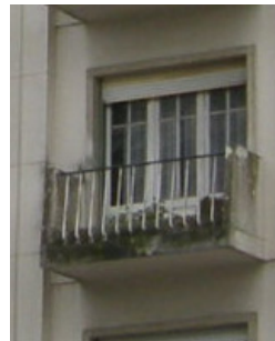
Figures 88 – Balconies (photos: SE 2010)
