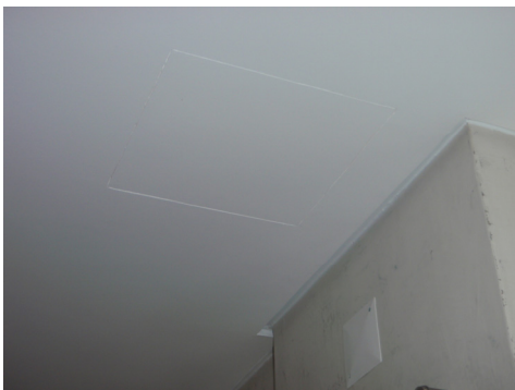
Figure 183 – Access hatch in plasterboard suspended ceiling in rehabilitated dwelling (photo: AC 2008)
