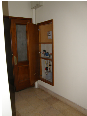
Figure 146 (left) – Set of meters in a ground floor room of a building (source: www.epul.pt )
