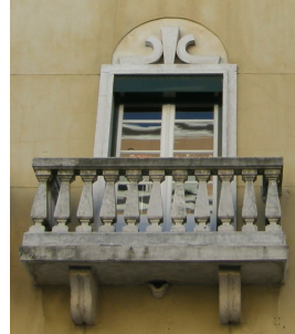
Figures 87 – Windows (photos: SE 2010)
