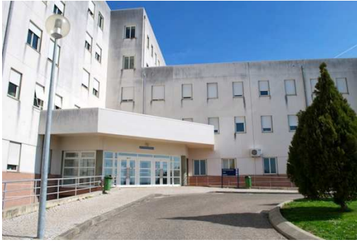
Figure 2.7 External space of the new G hospital
