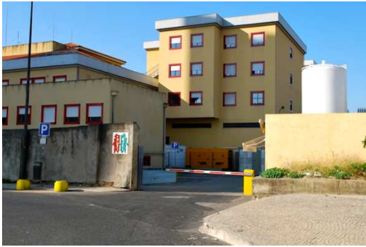
Figure 2.1 External space of the old G hospital
