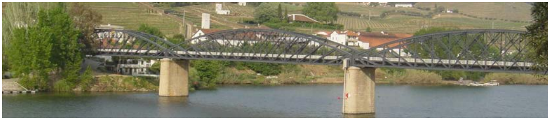
(a) Global view of Pinhão Bridge
