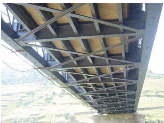
(d) View of bridge from below
