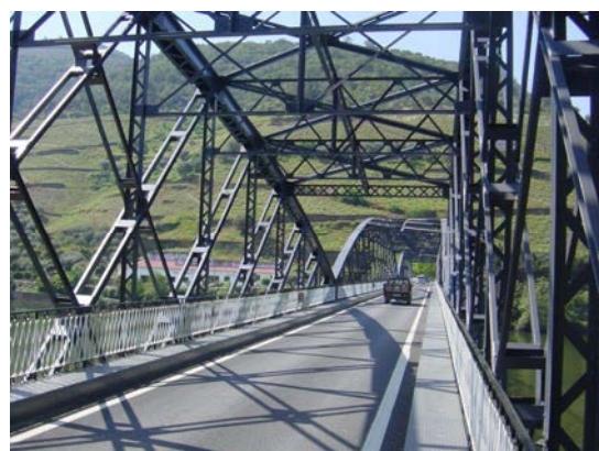
(e) View of bridge deck and select truss structure
