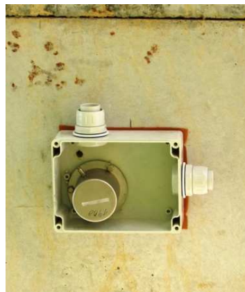
(a) Accelerometer installed at the bottom surface of the footbridge deck
