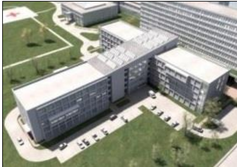
Figure 2.2 – Overview of the constructed building
