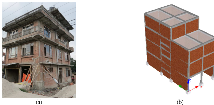
Figure 5.20 – CCP2 building; (a) Real building and (b) Numerical model
