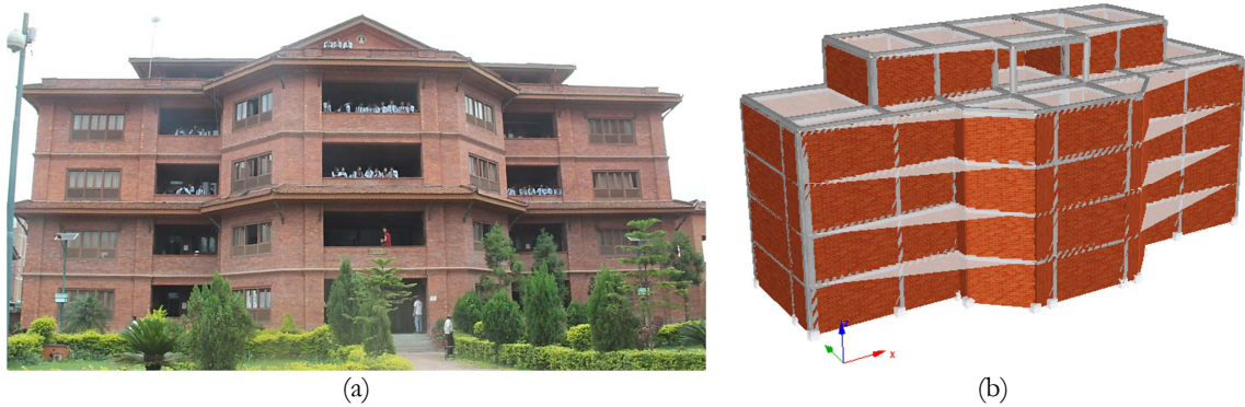
Figure 5.38 – WD1 building; (a) Real building and (b) Numerical model
