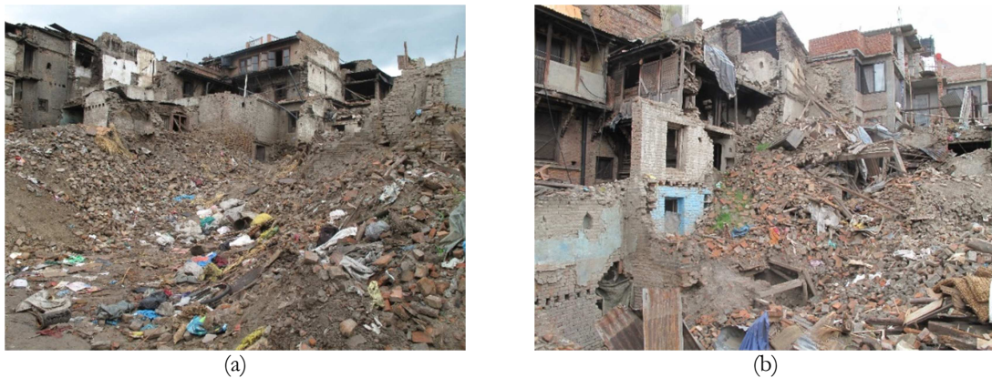
Figure 2.14 - URM earthquake damages and failure modes; (a) and (b) Partial or total collapse
