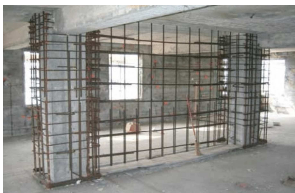
Figure 4. 29 – Shear wall constructed in the existing building
