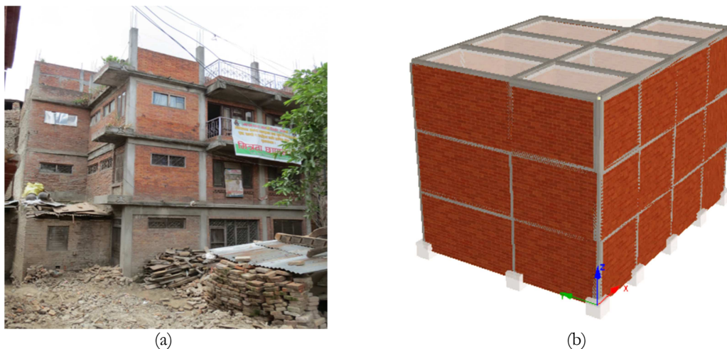
Figure 5.12 – CCP1 building; (a) Real building, and (b) Numerical model
