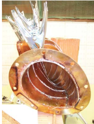
Fig. 7.16. Soldering the two halves from the interior of the vacuum vessel sector with Bi-Sn.
