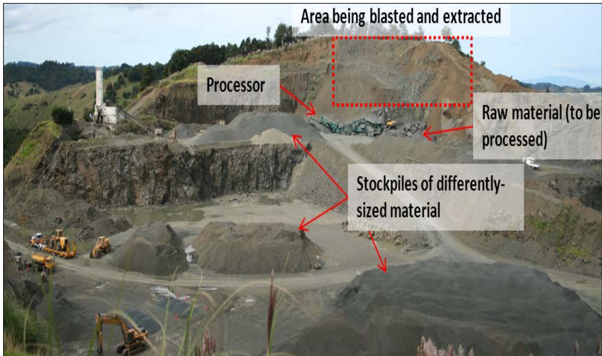
Figure 6.2 Flat Top quarry in New Zealand with typical features marked. The quarries at Bombay, Puketutu and Hunua (all New Zealand) shared these features and had a similar layout.
