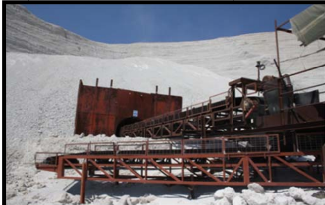
Pumice is dug from the wall and pushed by a front loader onto the roof of a tunnel
