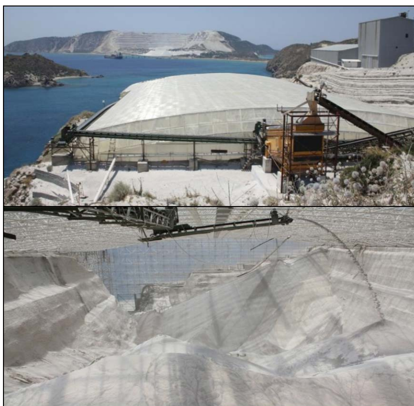
Figure 6.25 The perlite stockpile hangar on Yali which prevents raw perlite from exposure to rainfall.
