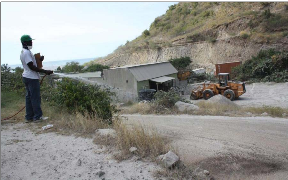
Figure 6.20 Spraying water with a hose to minimise the dust from the road from becoming re-suspended at Little Bay, Montserrat. Note the worker is wearing his respiratory protection on his chin.
