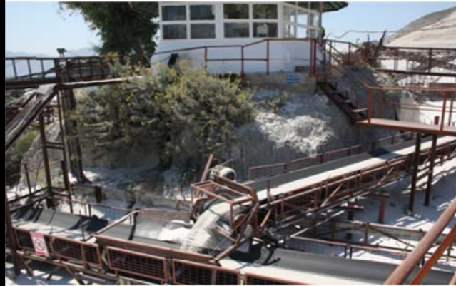
Processed material travels by conveyor belt either to a stockpile, or out to sea...
