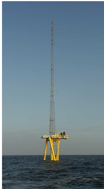
Figure 1.3: Demonstration of the IBGS at Hornsea [58].
