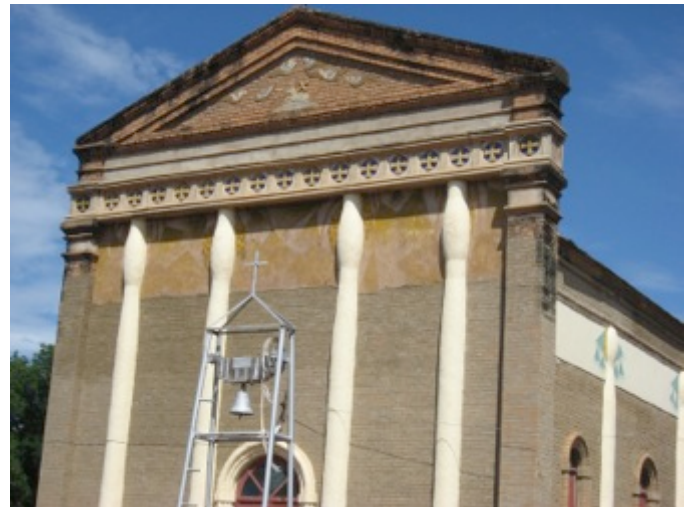
Image 59 Detail of re-roofed Kuajok Church, 2011 note: palm trees on side walls are repainted
