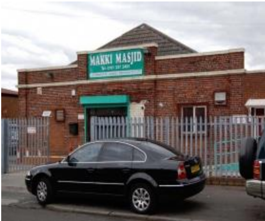
Figure 5.15 The old Makki Masjid in a redundant cooperative shop
