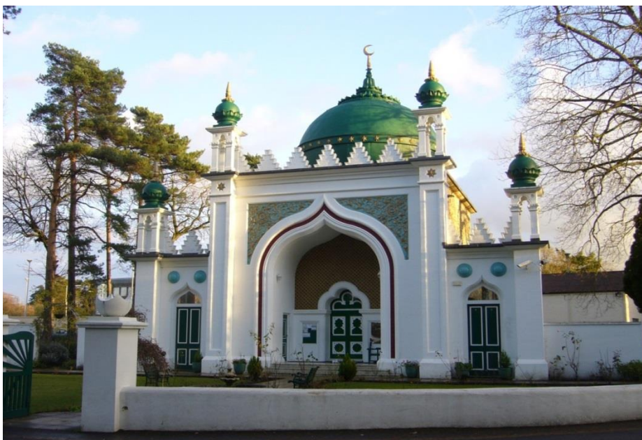
Figure 5.2 Shah Jahan Mosque in Woking - First fully functional purpose built mosque in Britain established in 1889.
